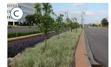
Rain garden + tree trench
