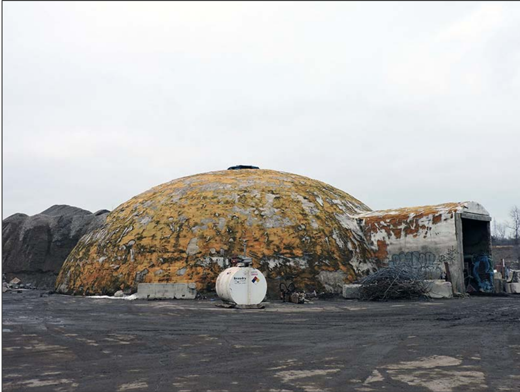
Figure 19. Monolithic Dome (HE-MPC-9263), Facing Northeast
