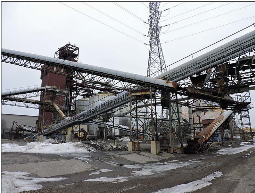
Figure 12. Conveyors (HE-MPC-9257), Facing Northwest
