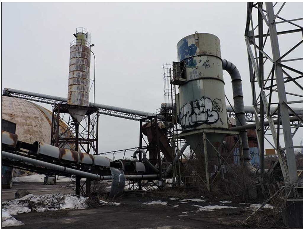
Figure 15. Dust Collection Tank and Storage Tank (HE-MPC-9262), Facing Northeast
