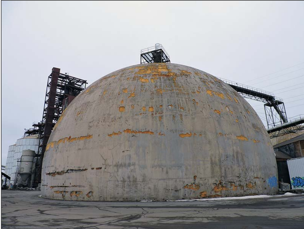
Figure 26. Monolithic Dome (HE-MPC-9266), Facing Northeast
