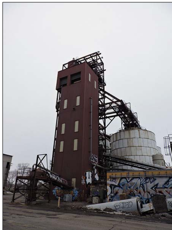
Figure 14. Grain Elevator (HE-MPC-9259), Facing Northwest
