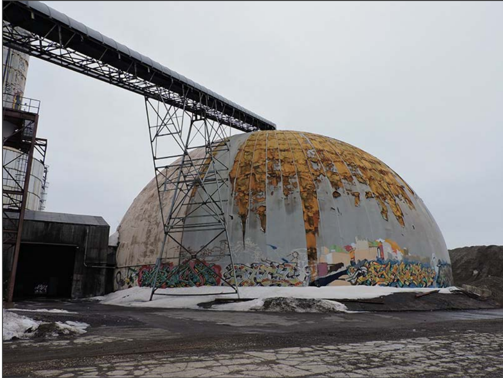
Figure 21. Monolithic Dome (HE-MPC-9264), Facing Northwest
