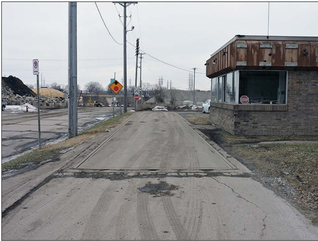
Figure 10. Scale House (HE-MPC-9245) and Truck Scale (HE-MPC-9246), Facing East
