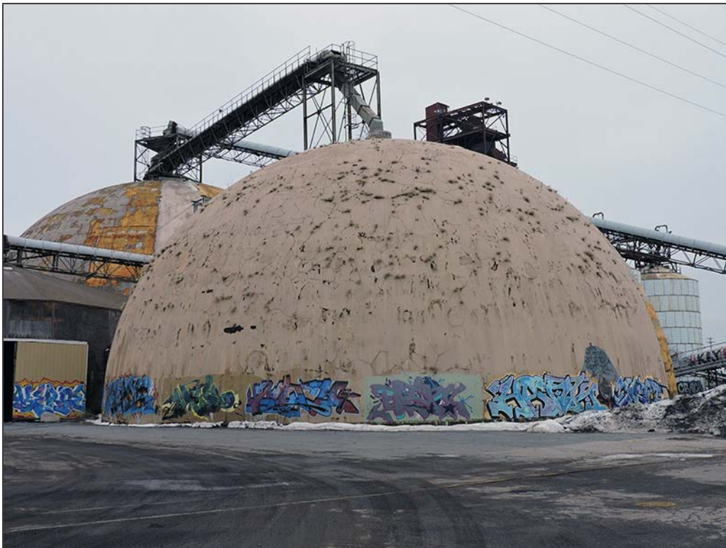
Figure 23. Monolithic Dome (HE-MPC-9265), Facing Northwest
