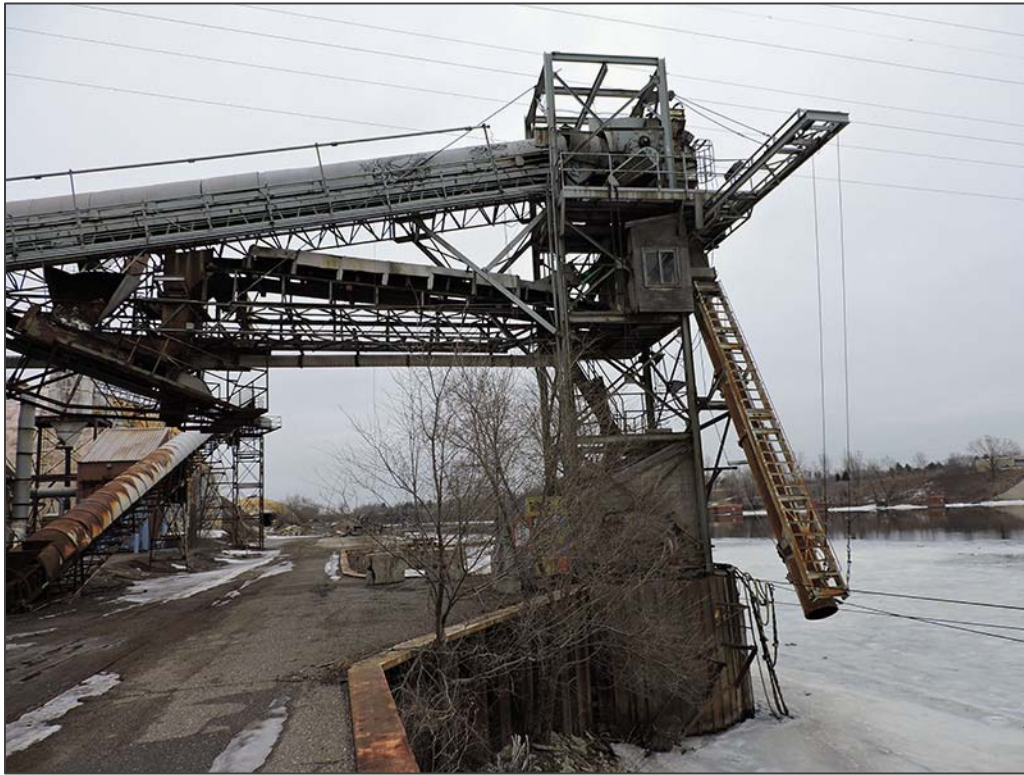
Figure 13. Load-out Tower (HE-MPC-9256), Facing North
