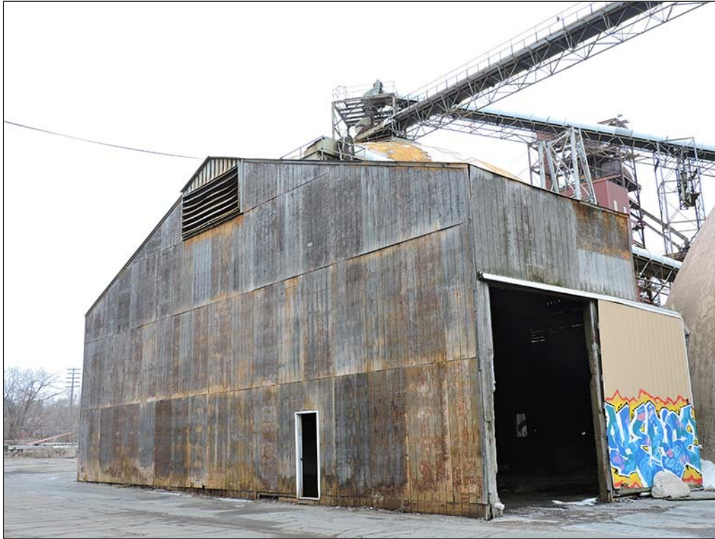
Figure 17. Load-out Shelter (HE-MPC-9268), Facing Northwest
