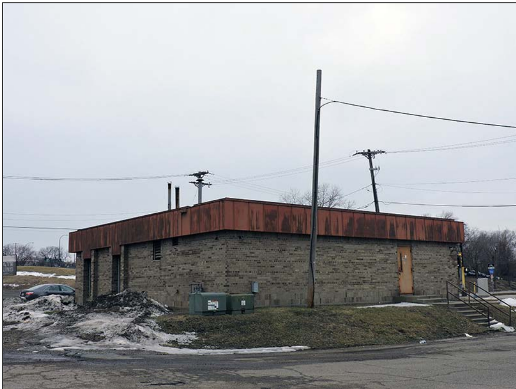
Figure 9. Office Building (HE-MPC-9244), Facing NW
