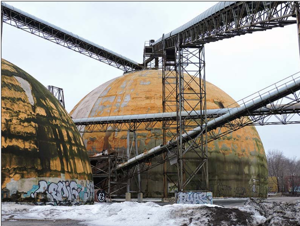
Figure 25. Monolithic Dome (HE-MPC-9266), Facing Southwest
