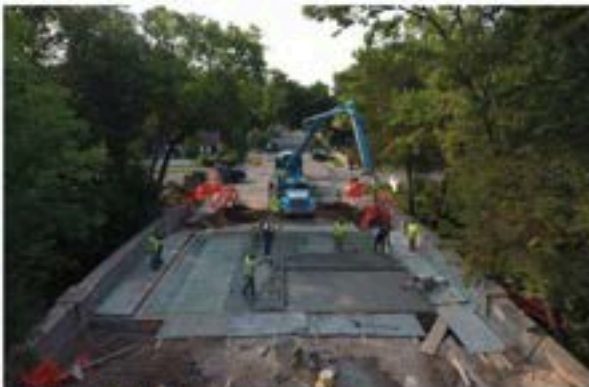
Bridge repair and rehabilitation underway
