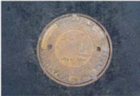
Manhole Cover Replacement
