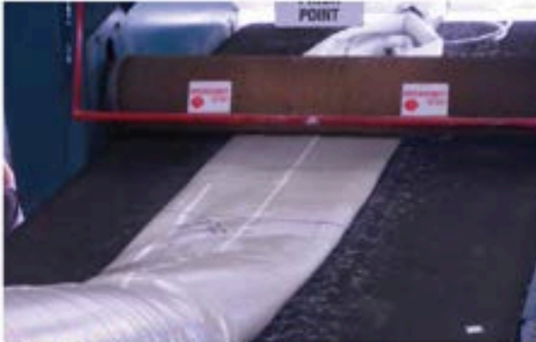
Cured-in-Place Pipe Lining
