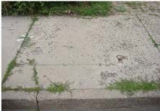
Deteriorated Sidewalk
