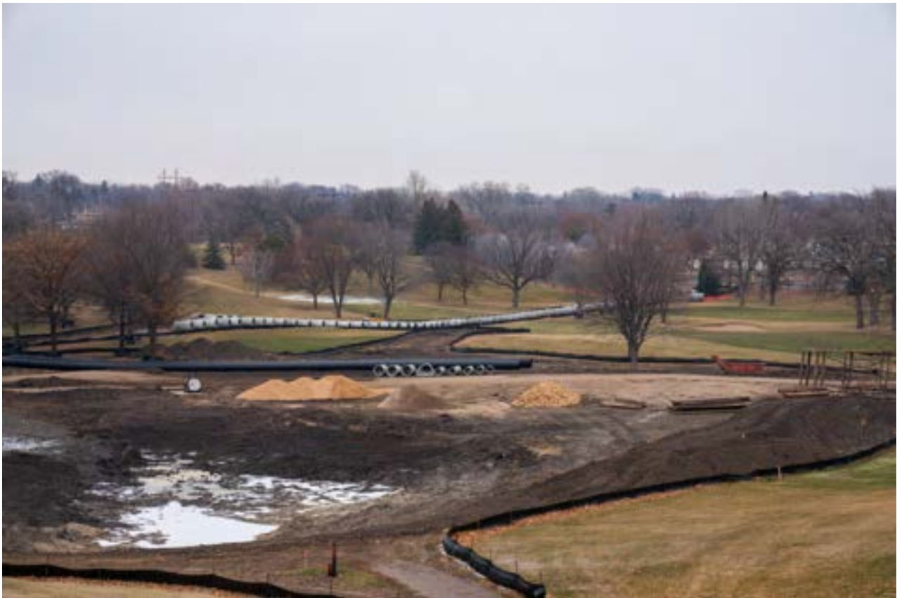
Recent construction of infiltration basin and larger storm sewers at the Columbia Golf Course
