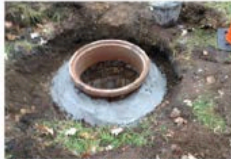
Infiltration & Inflow Repairs
