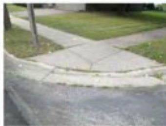
Some pedestrian ramps do not meet current ADA standards for accessibility.
