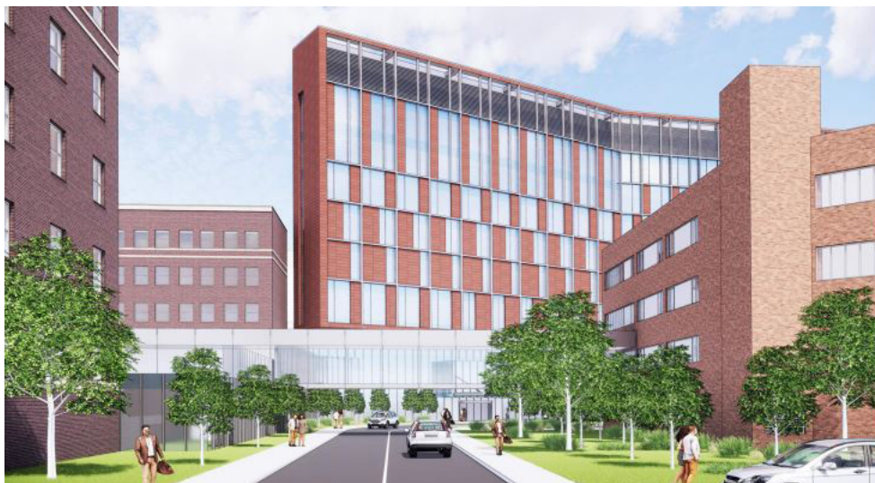
Allina Care Pavilion (Credit: HGA)
