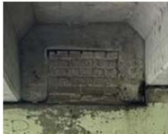
Filled utility blockout
