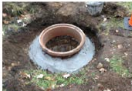
Infiltration & Inflow Repairs
