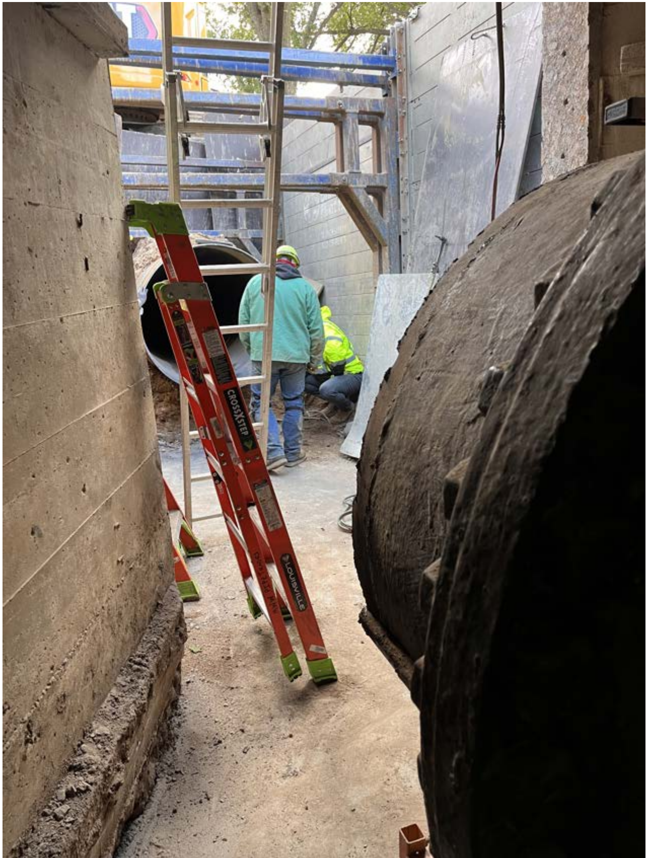
Performing a repair in a large valve chamber and transmission main.
