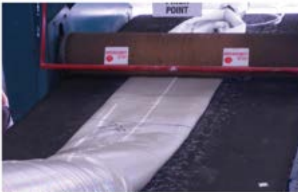
Cured-in-Place Pipe Lining
