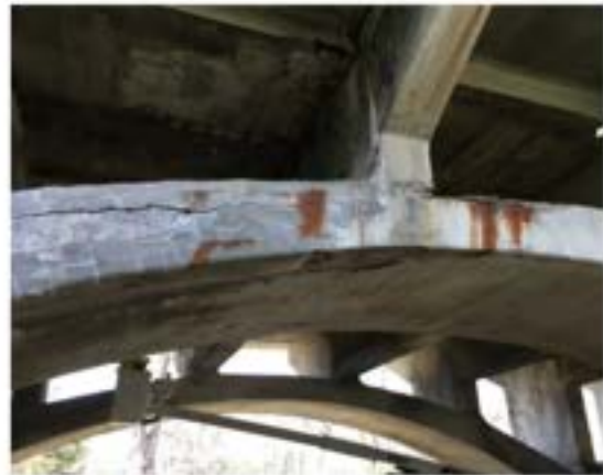
Major Crack & Concrete Deterioration on Arch Rib
