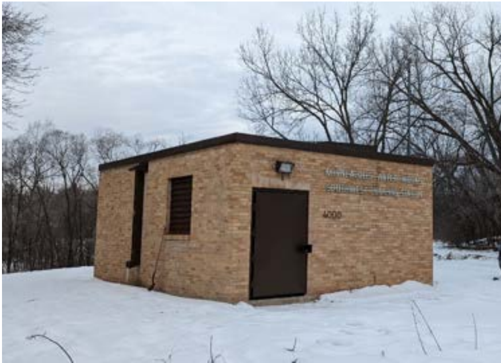
Photo of the existing SouthWest Pump Station.
