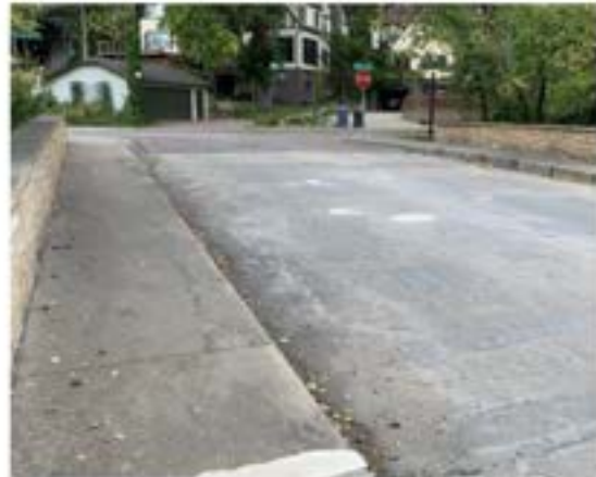
Deck Patching and joint repair
