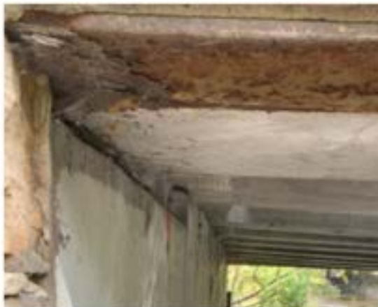
Steel lintel at north abutment
