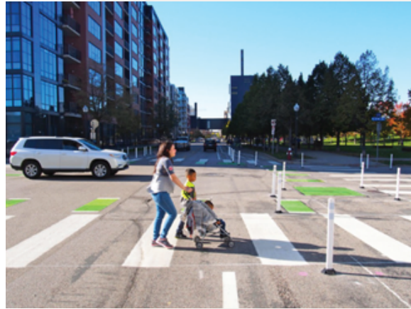
Delineator-protected bikeways use plastic delineator posts or “bollards” and a painted buffer space between the bikeway and the travel or parking lane to provide physical separation from motorized traffic. Photo: delineator-protected bikeway along 2nd Street S.
