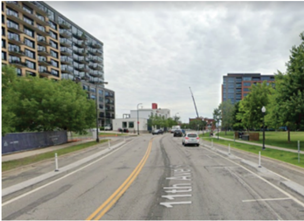
Curb-protected bikeways use a form-in-place concrete curb installed on the roadway surface to provide physical separation from traffic. Photo: curb-protected bikeway along 11th Avenue S.
