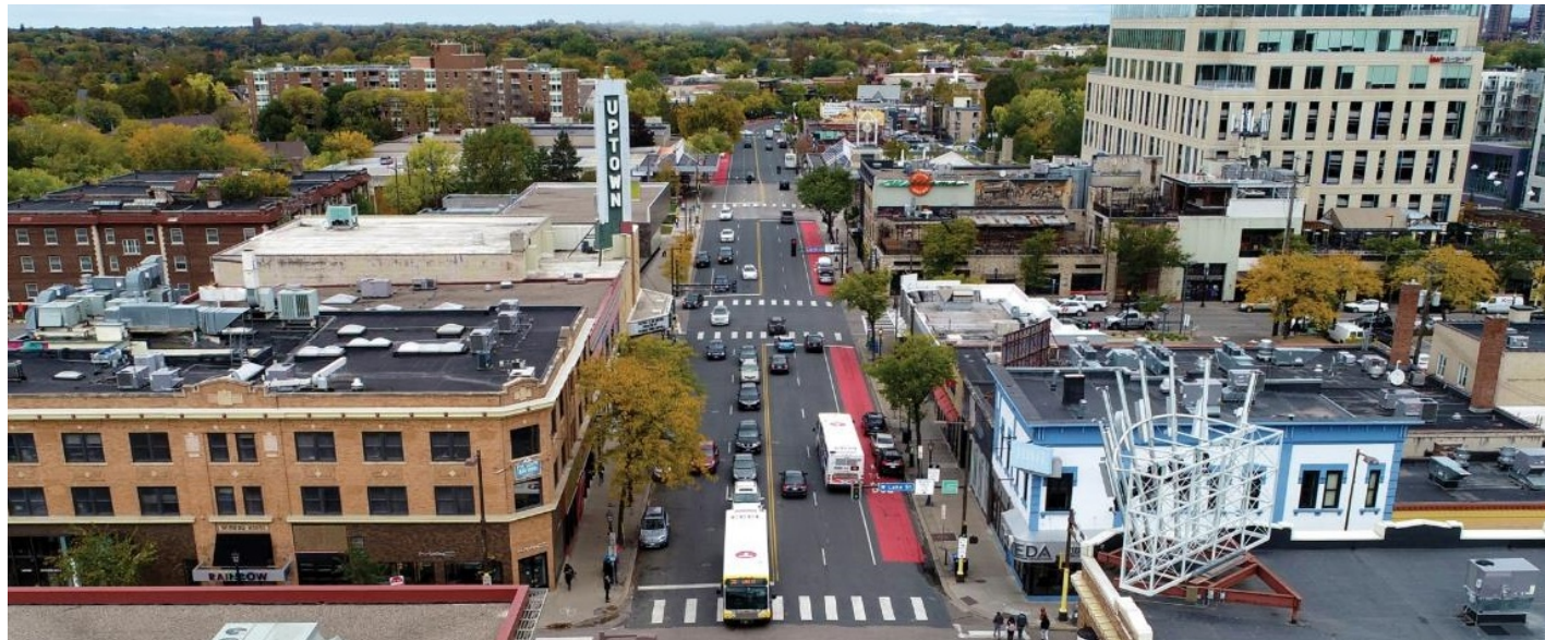
Existing bus lanes on Hennepin Avenue north of Lake Street
