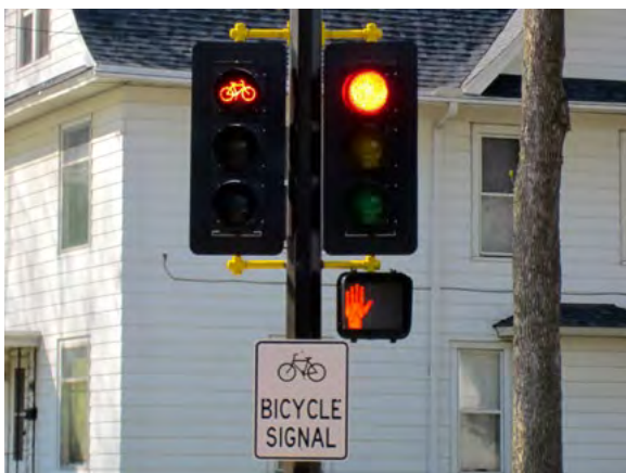
Figure 8-8: 12-inch signal heads and “Bicycle Signal” signing on southbound 5 th Street Northeast approach at Broadway Street Northeast after installation
