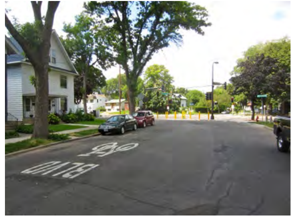
Figure 8-5: 5 th Street Northeast approaching Broadway Street Northeast from the south after installation*
