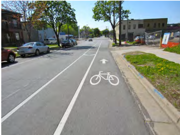
Figure 14-4: Fremont Avenue North approaching West Broadway Avenue North after installation
