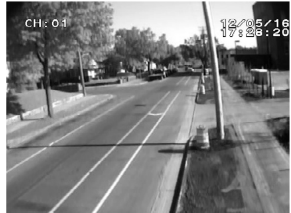
Figure 14-9: Screen capture of after video on Fremont Avenue North between 21 st Avenue North and 22 nd Avenue North
