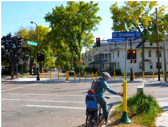
Figure 8-6: Southbound bicyclist and passenger actuating the bicycle phase to cross Broadway Street Northeast after installation
