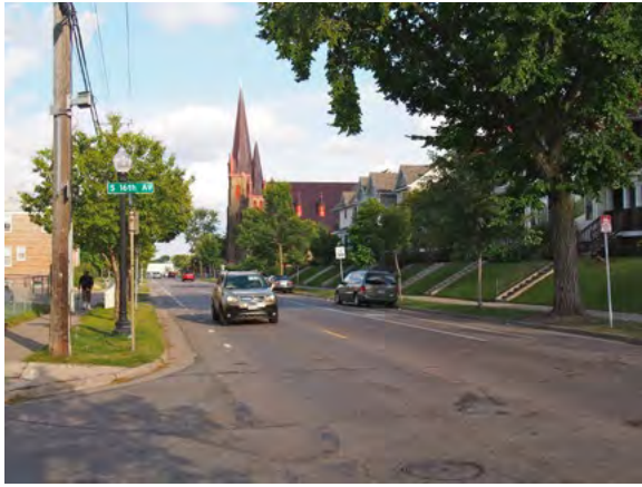
Figure 10-3: 24 th Street East facing west at 16 th Avenue South after installation
