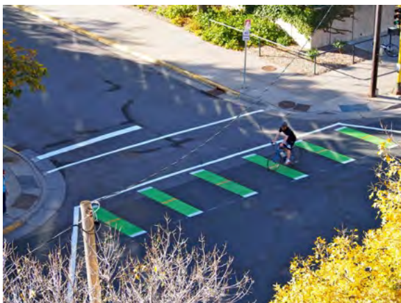
Figure 4-12: Example of modified dotted green conflict zone installed parallel to a crosswalk
