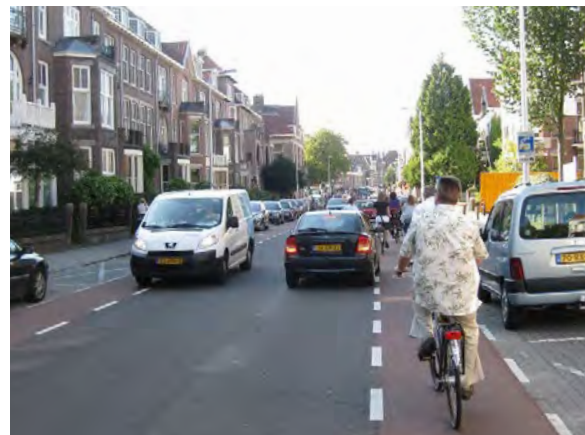
Figure 7-4: Example of two oncoming motorists negotiating on a street with advisory bicycle lanes in Utrecht, Netherlands
