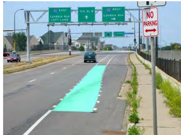
Figure 3-4: 7 th Street North at East Lyndale Avenue North facing northwest after installation
