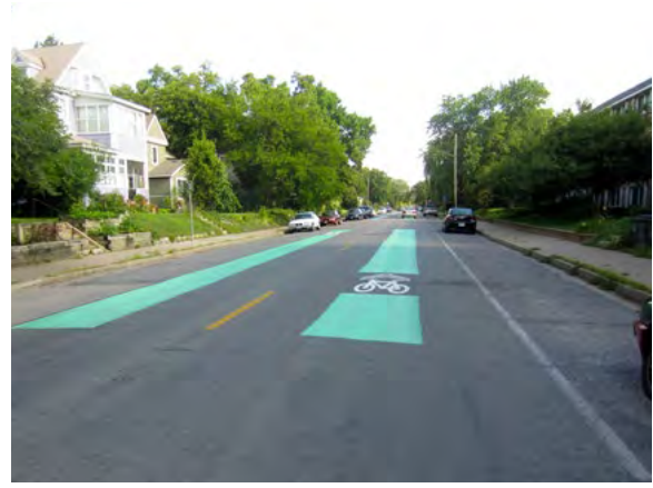
Figure 6-6: Bryant Avenue South facing north at 35 th Street West after installation with updated intermittent colored background for shared lane markings
