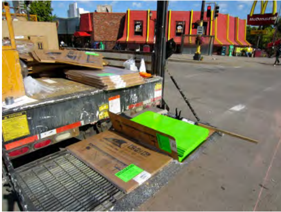
Figure 16-7: Preformed thermoplastic material panels prior to installation
