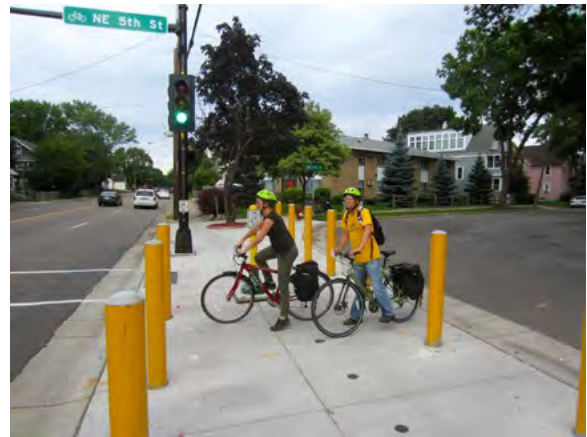
Figure 8-7: Two northbound bicyclists waiting for the green bicycle phase to cross Broadway Street Northeast after installation
