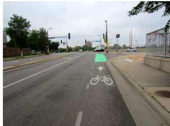
Figure 3-7: 16 th Street East at 3 rd Avenue South (eastbound) facing east after installation
