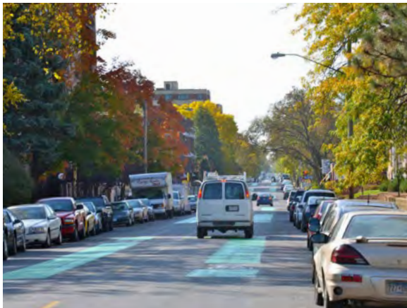
Figure 6-9: Motor vehicle traveling south on Bryant Avenue South at 35 th Street West after installation
