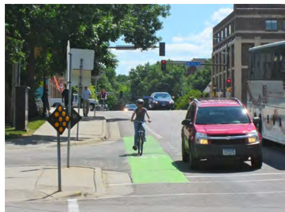
Figure 16-6: Bicyclist riding northbound on 15 th Avenue Southeast at 5 th Street Southeast after installation
