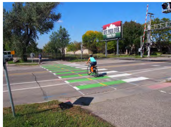
Figure 4-13: Example of modified dotted green conflict zone installed parallel to a crosswalk
