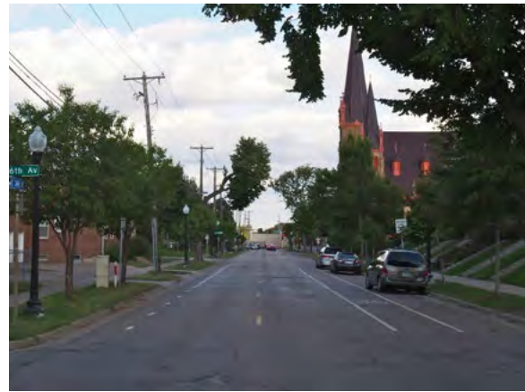
Figure 10-6: 24 th Street East facing east at 16 th Avenue South after installation
