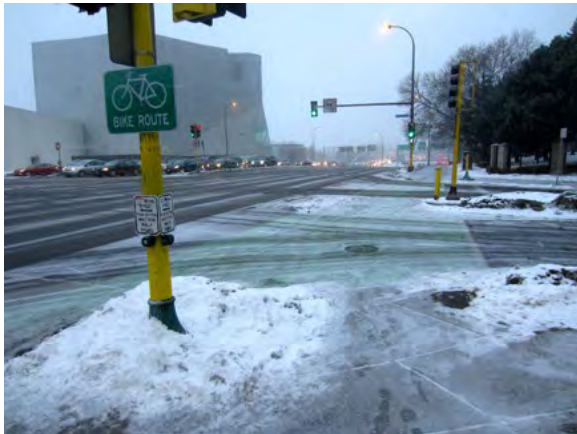
Figure 2-1: Snow limits the visibility of a colored crosswalk on Hennepin Avenue South at Groveland Avenue South
