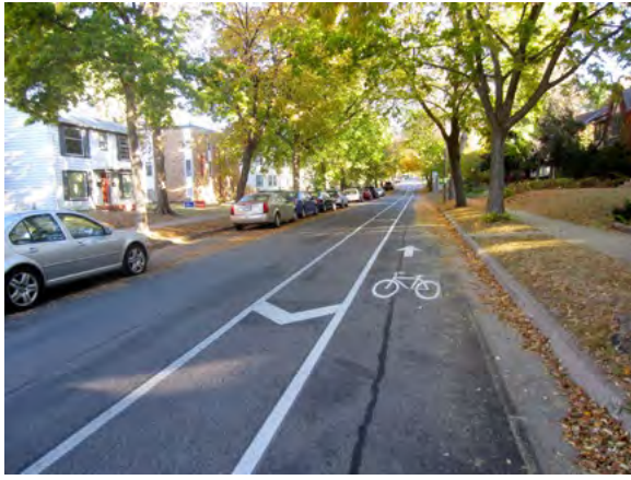
Figure 15-4: 1 st Avenue South at 39 th Street East after installation on a weekday
