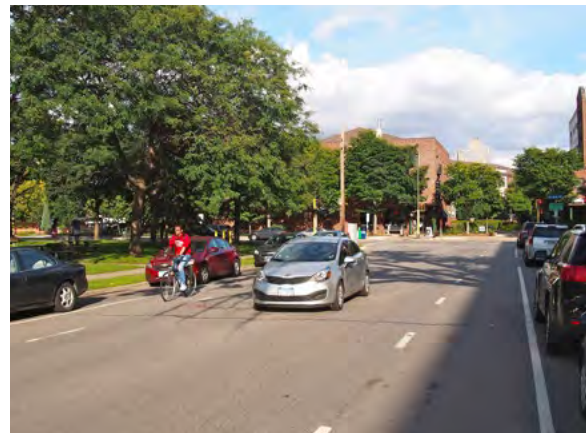
Figure 7-12: A bicyclist and motorist traveling on 14 th Street East facing east towards 11 th Avenue South after installation with a 18-foot two-way travel lane after installation
