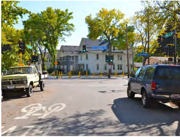
Figure 8-4: 5 th Street Northeast approaching Broadway Street Northeast from the north after installation
