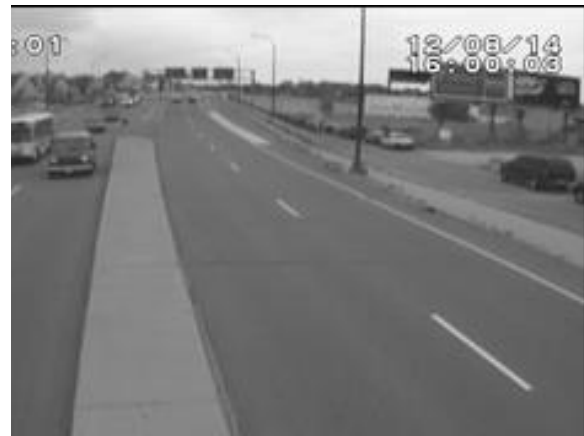
Figure 3-13: Screen capture of after video of 7 th Street North between 10 th Avenue North and East Lyndale Avenue North
