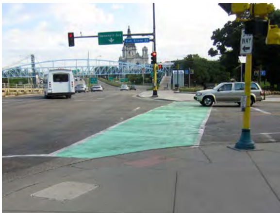
Figure 4-6: Oak Grove Street West intersection after installation with updated colored crosswalk
