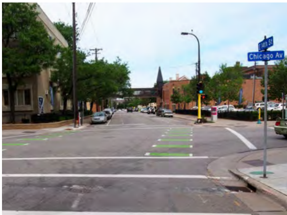
Figure 7-11: 14 th Street East facing east at Chicago Avenue South after installation at the transition from a 14-foot to 18-foot two-way travel lane
