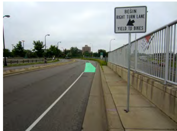
Figure 3-9: 16 th Street East at I-94 westbound on-ramp facing east after installation
