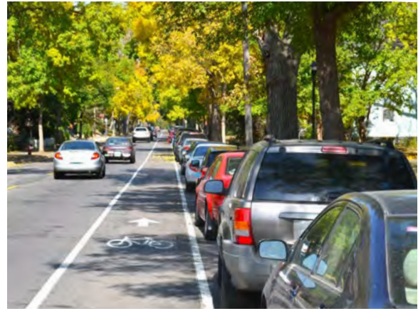
Figure 13-4: Traffic on 1 st Avenue South at 25 th Street East after installation
