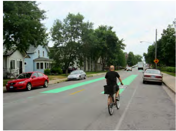
Figure 6-8: Bicyclist riding south on Bryant Avenue South at 38 th Street West after installation
