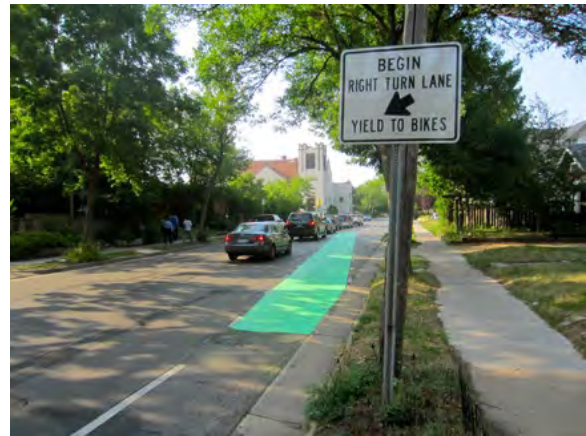
Figure 3-10: 1 st Avenue South at 28 th Street East facing north after installation
