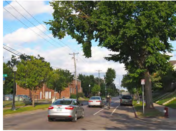
Figure 10-4: 24 th Street East facing east at 16 th Avenue South after installation
