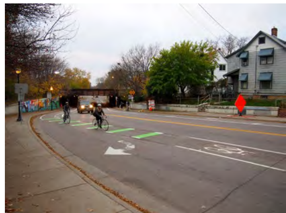
Figure 3-15: Example of modified dotted green conflict zone at a developing right turn lane
