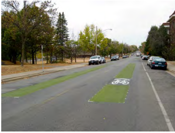
Figure 6-5: Bryant Avenue South facing north at 40 th Street West in 2011 after installation with original intermittent colored background for shared lane markings
