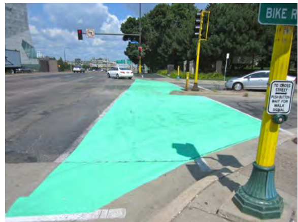
Figure 4-7: Groveland Avenue South intersection after installation with updated colored crosswalk
