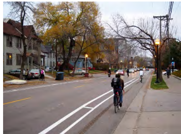
Figure 17-7: Buffered bicycle lane between 5 th Street Southeast and 6 th Street Southeast in 2015
