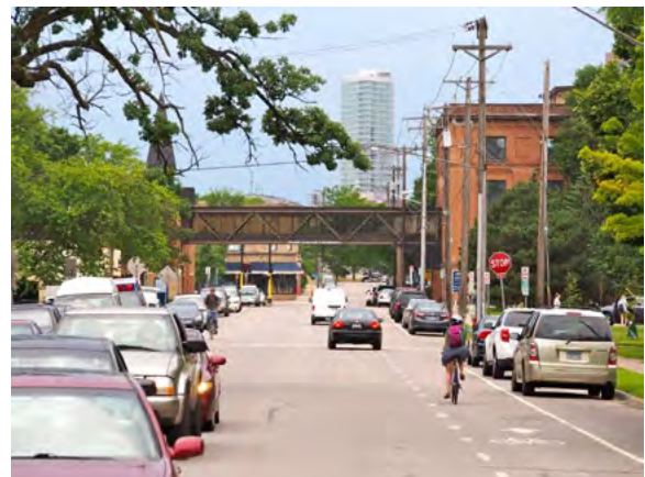
Figure 7-14: Traffic on 14 th Street East between 11 th Avenue South and Elliot Avenue South after installation with a 18-foot two-way travel lane
