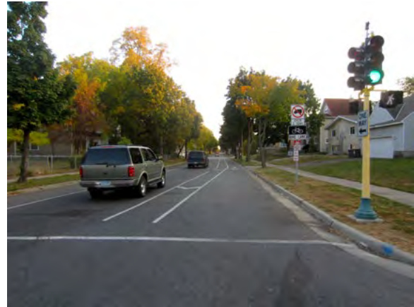
Figure 14-5: Traffic on Fremont Avenue North at 26 th Avenue North after installation
