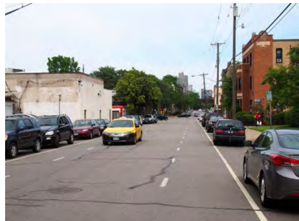
Figure 7-8: 14 th Street East facing east at Park Avenue South after installation with a 14-foot two-way travel lane
