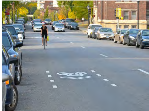
Figure 5-6: A southbound bicyclist on LaSalle Avenue South at Groveland Avenue South after installation
