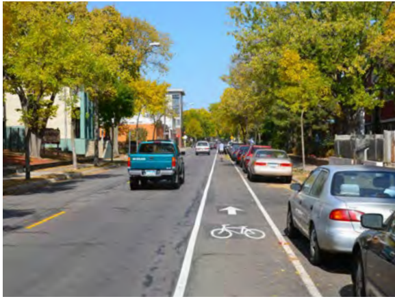
Figure 13-3: 1 st Avenue South at 27 th Street East after installation
