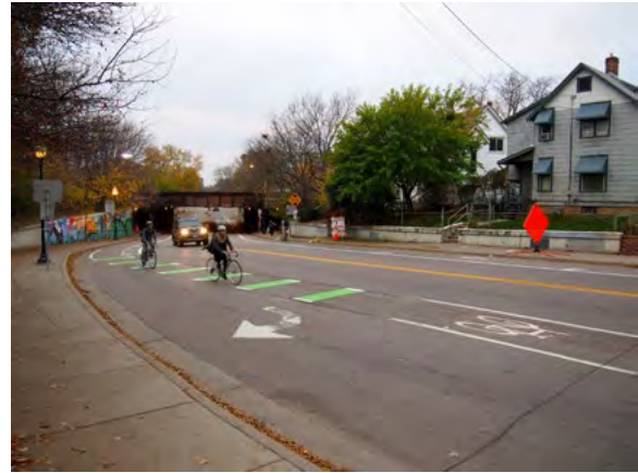
Figure 16-14: Example of modified dotted green conflict zone at a developing right turn lane
