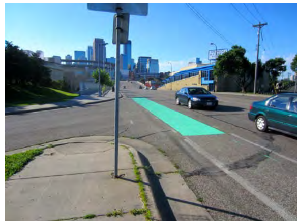
Figure 3-5: 7 th Street North at 6 th Avenue North facing southeast after installation
