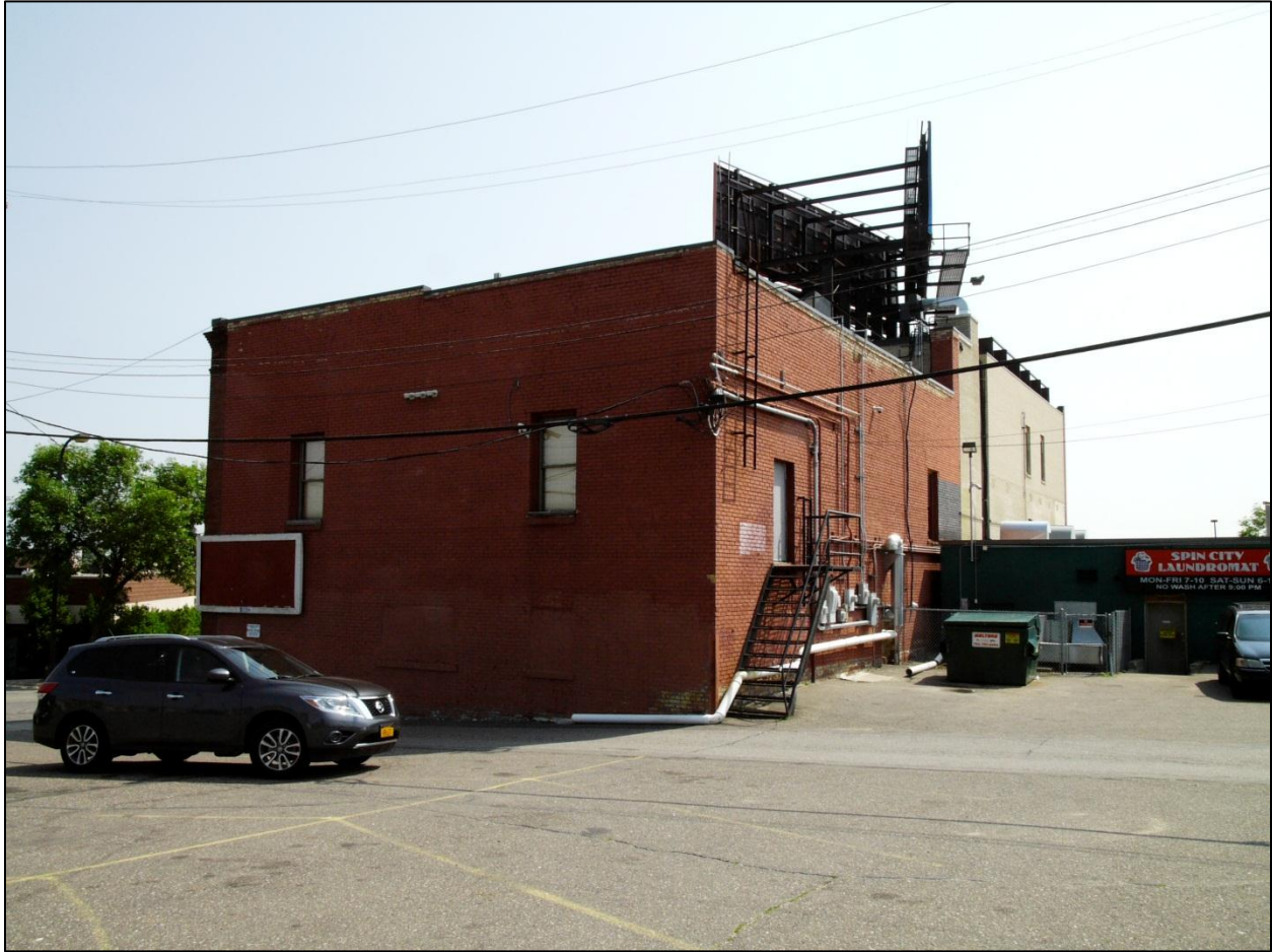
Figure 7. Secondary elevations, historic cream colored brick has been painted over, note infilled windows. Source: CPED files.
