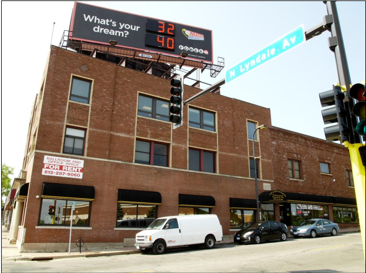
Figure 6. 42 nd Avenue North Frontage, note the billboard, the missing crenelated parapets and the storefront alterations. Source: CPED files.
