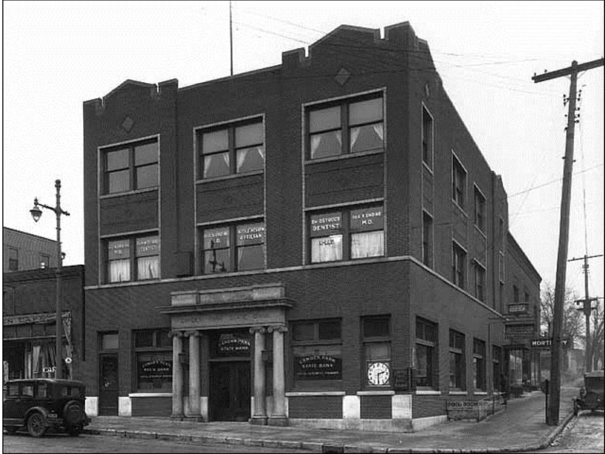
Figure 1. Camden Park State Bank 1920s, Lyndale Avenue frontage. These are the primary elevations. Note the main entry portico, the windows, the crenelated parapets, the signage, the flagpole, the clock, and the basement level entry along 42 nd Avenue North. Source: Minnesota Historical Society.
