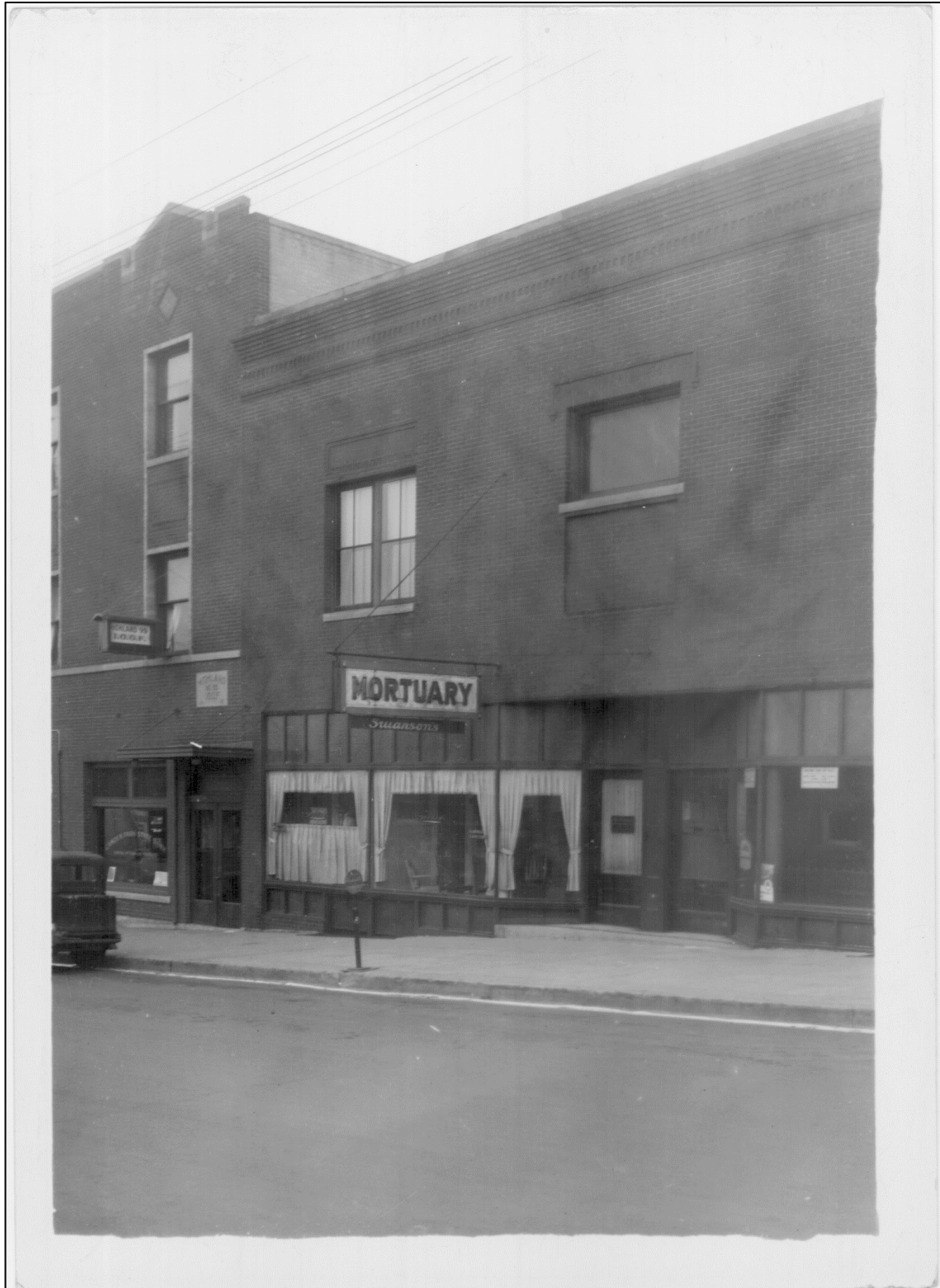
Figure 2. Camden Park State Bank Building, 1938. 42 nd Avenue North frontage. Any alteration of the storefront to the 1910 building should move towards a restoration dating to the period of significance. Note the signage, the rain screen over the double door entry to the ballroom and the crenelated parapets. Source: Minnesota Historical Society.
