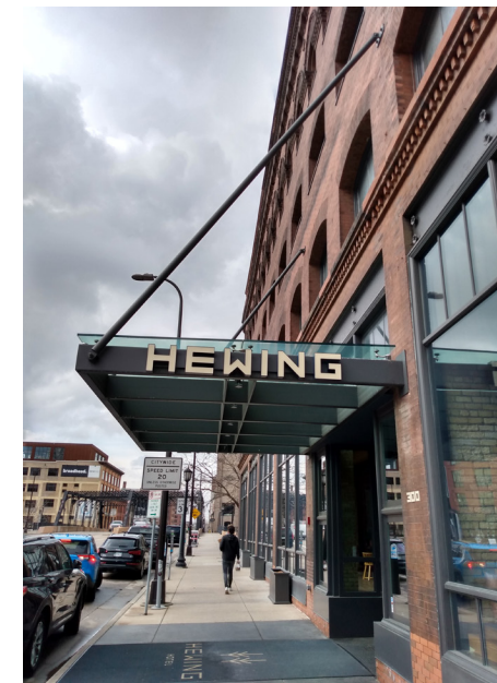
Signs may be mounted to the fascia of canopies, provided the letters do not extend above or below the fascia.
