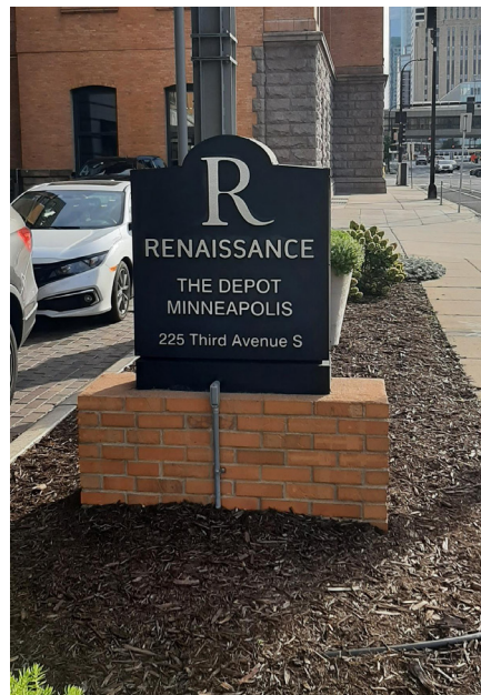
Freestanding signs should be constructed of materials similar to those found on the existing building or compatible with the existing building, like the brick and dark colored aluminum found in this sign and its historic building.
