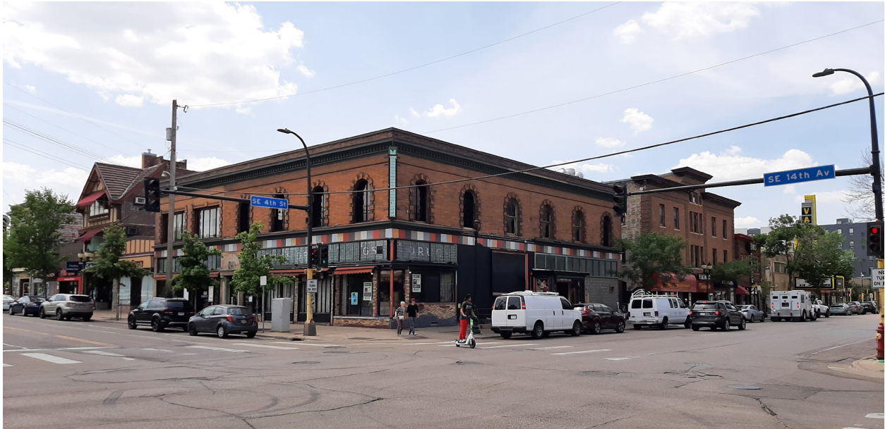
Dinkytown Commercial Historic District at 4th St SE and 14th Ave SE, looking west.
