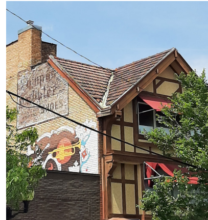
Look at the details on 321 14th Ave SE, built in 1910. The primary elevation has half-timbering and wood brackets under the eaves. The roof is covered with terracotta tiles. The side elevation has a ghost sign for a previous tenant and a colorful mural.
