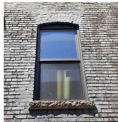
This window has a brick arch above and a stone sill below. Lintels, pediments, moldings, and hoods are typically found around the tops of windows.
