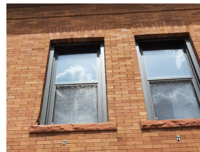
These replacement metal windows at 1401-1411 4th St SE are set within the historic openings. The jack arches above and sills below are original.
