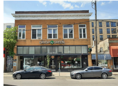
411-413 14th Ave SE, built in 1904, is a contributing resource.
