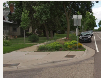
Curb extensions to reduce pedestrian crossing distance
