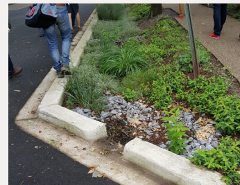
Bioretention curb extensions
