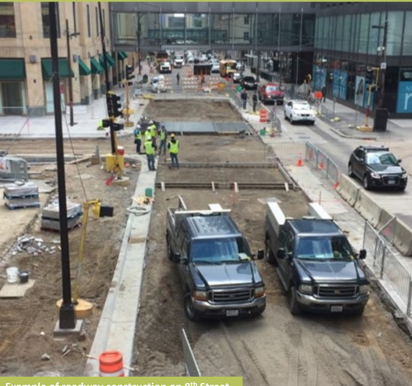
Example of roadway construction on 8 th Street
