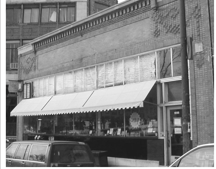
Retain and rehabilitate historic storefronts, including transoms, sidelights, and display windows.
