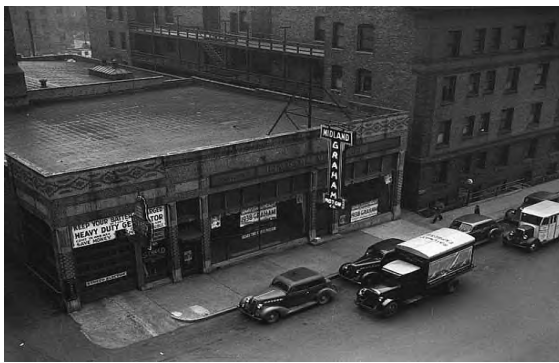
A 1937 rooftop view of the building housing the Streed Electric Co. and the Midland (Graham) Motor Co. at 1317 Harmon Place shows the flat roof typical of most in the district, and the decorative brick parapet. (Photo: MHS)
