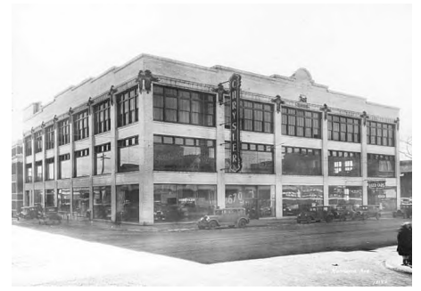
F.E. Murphy Auto Co. (1912-13), 1301 Hennepin Avenue. Reinforced concrete construction allowed the auto showroom walls to be filled with large display windows.
