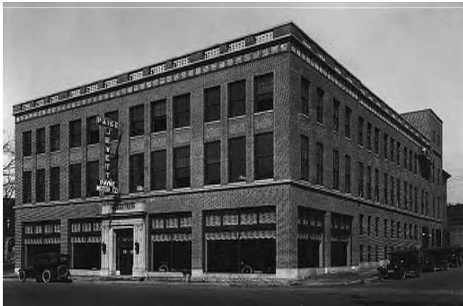
The Payne Motor Company (1916) at 1400 Harmon Place. The now-raised building showed the standard treatment of the large, three-story automotive building. The first floor was devoted to display, with storage and offices above. The elevator and service area is at rear. (Photo: MHS)
