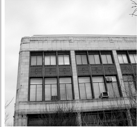
The ongoing settlement of the Loring Park area is evident on some building exteriors.
