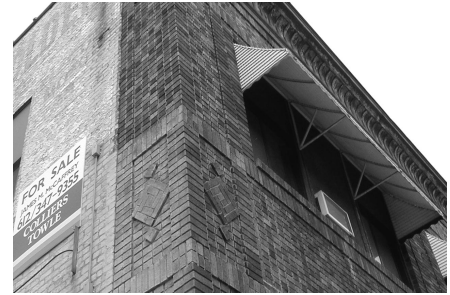
A decorative sheet metal cornice and brick panels at 1208 Harmon Place (1914).
