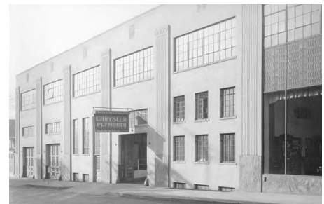
A variety of metal casement windows were used at the rear of many buildings in the district. (Photo: MHS)
