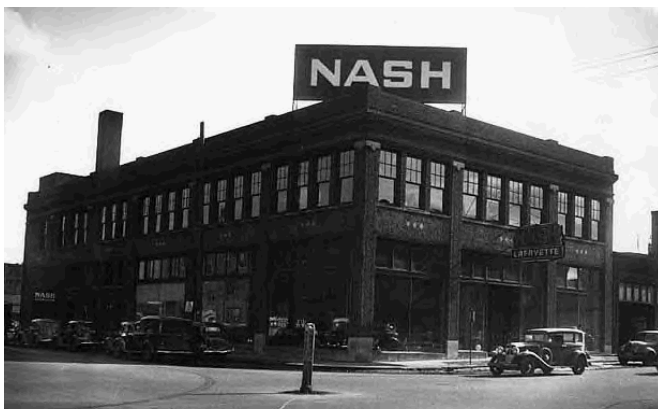
1201 Harmon Place (1920) in 1937 when it was the Northwest Nash Motor Company. The two-story building has simple geometric trim and large display windows that fill the bays at the street level. Above, the bays are filled with double-hung sash with divided lights. (Photo: MHS)
