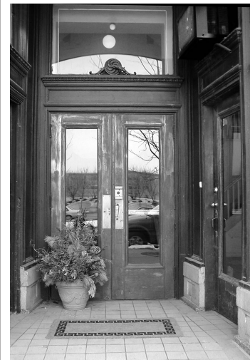
This deeply recessed entrance at the Fawkes Block retains many original features including a glazed transom over the double-leaf doors.
