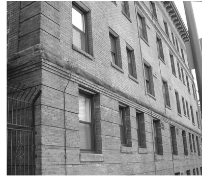
Conserve historic windows if possible and install compatible replacements only if necessary.
