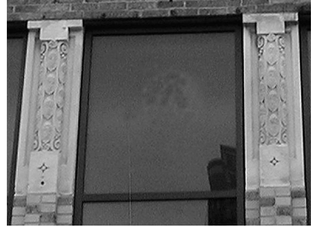
Terra cotta frames the windows at 1315-1317 Harmon Place (1923).
