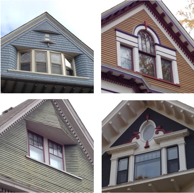
Fanciful dormers, decorative window detailing and Palladian windows. Note the treatment of the eave conditions.
