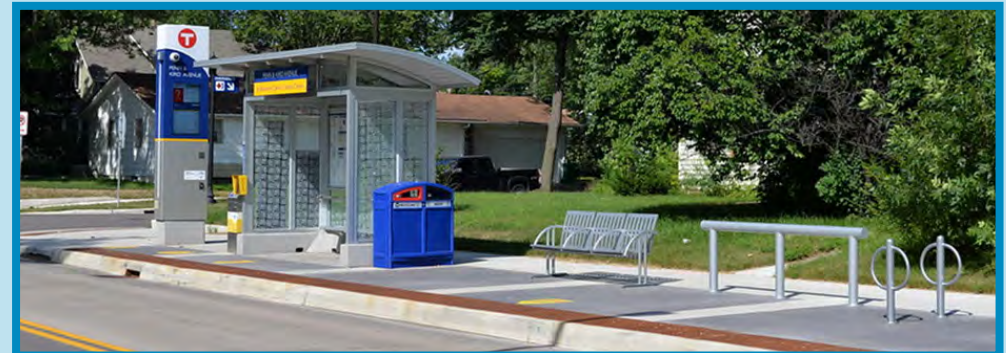
C Line BRT station platform
