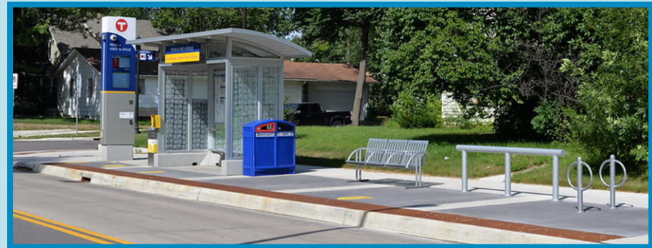
C Line BRT station platform
