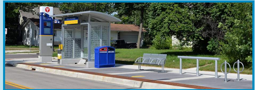
C Line BRT station platform
