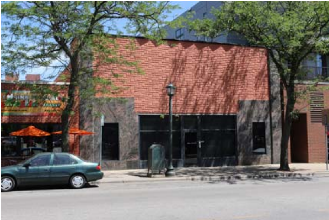
HE-MPC-16785, June 2018, primary facade, looking east
