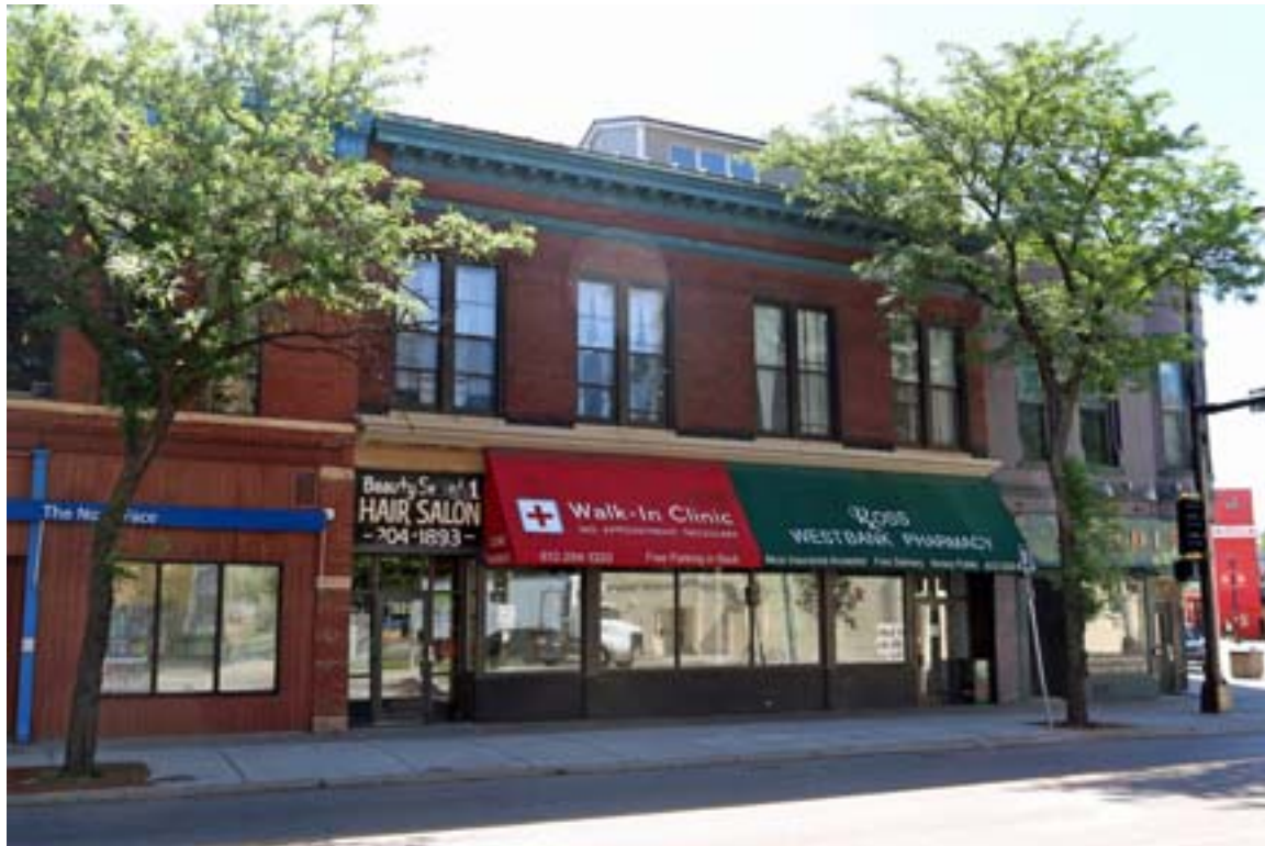
HE-MPC-4929, June 2018, front facade, looking east
