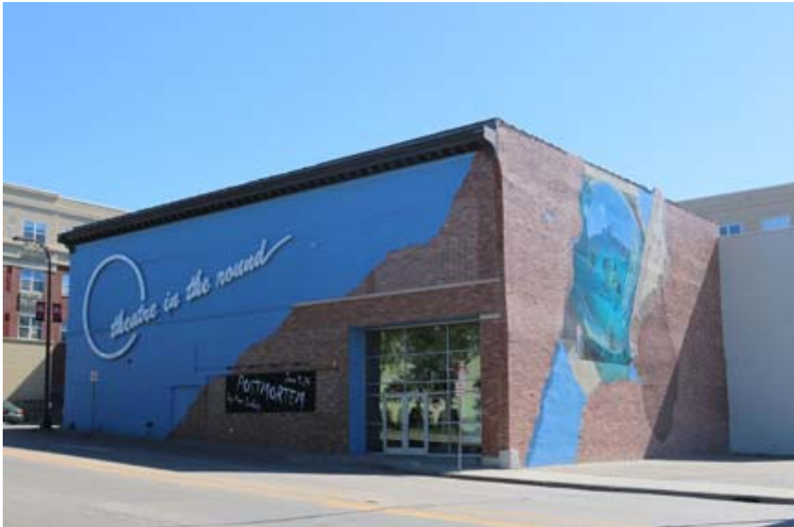
HE-MPC-19322, June 2018, front and south facades, looking northeast
