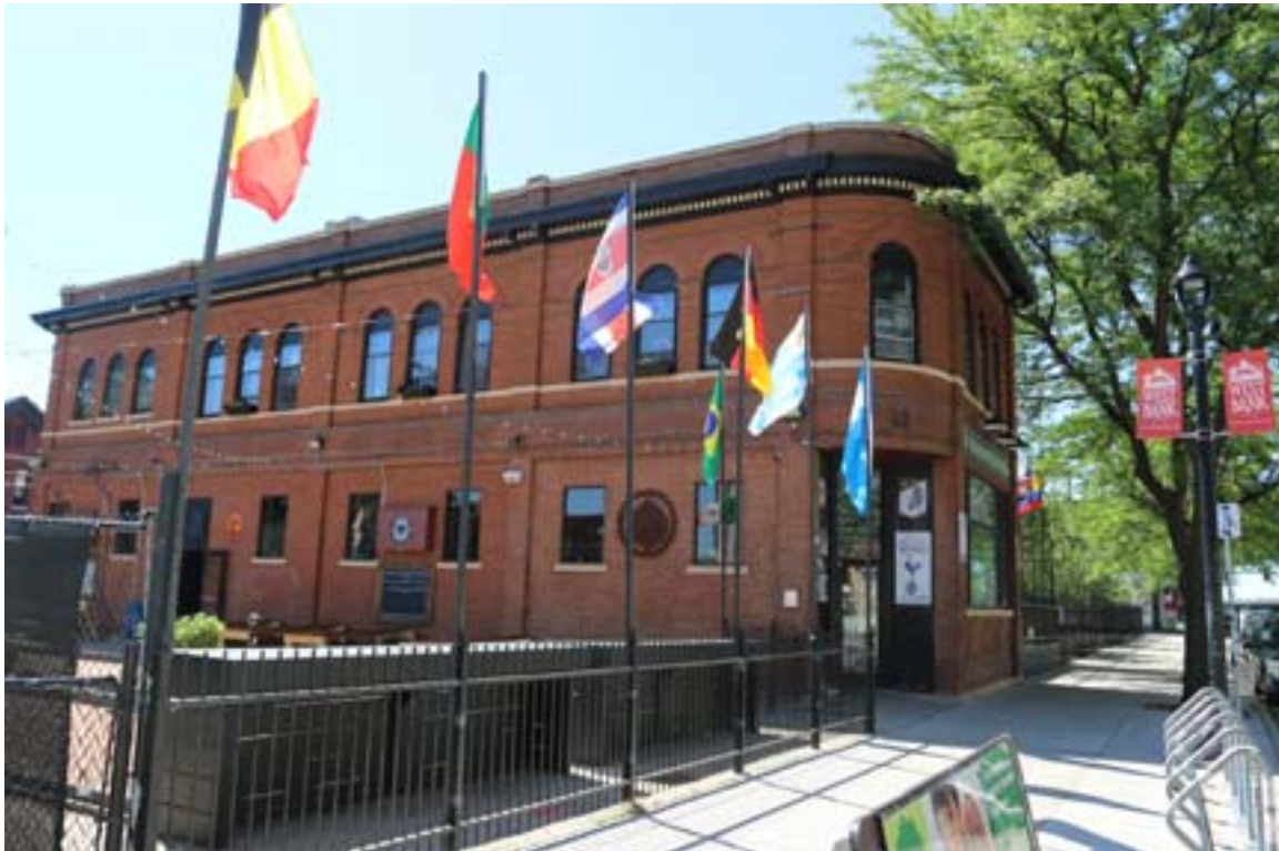
HE-MPC-4930, June 2018, primary facade, looking southeast
