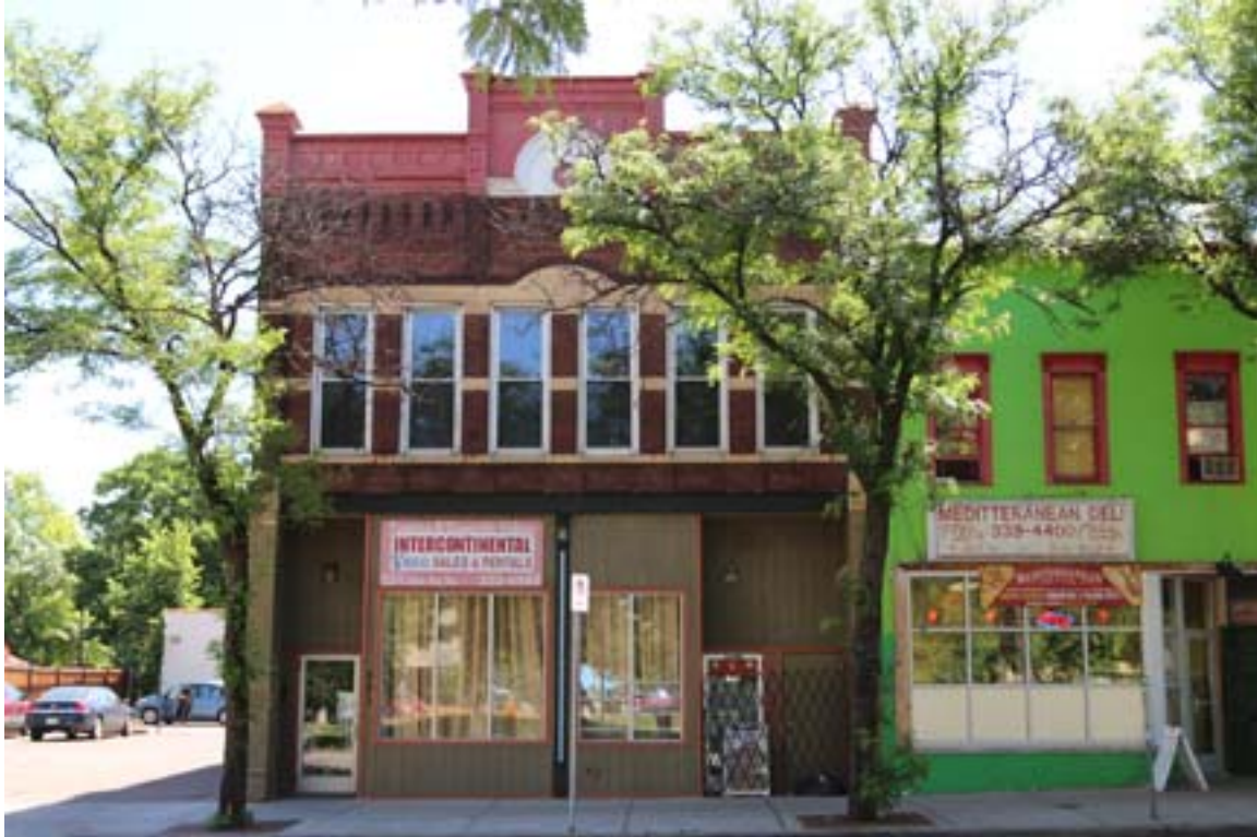
HE-MPC-4931, June 2018, primary facade, looking east
