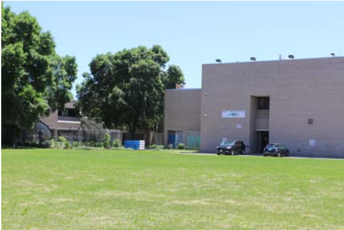
HE-MPC-8160, June 2018, primary facade, looking southeast
