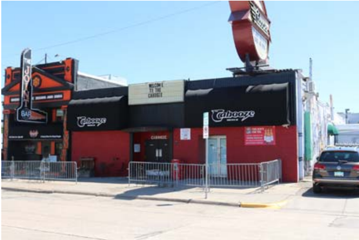
HE-MPC-19116, June 2018, primary facade, looking east
