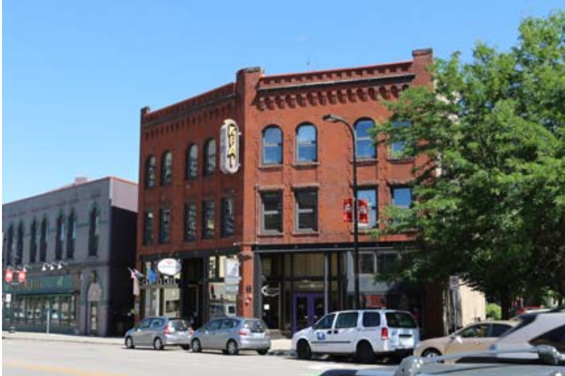
HE-MPC-4924, June 2018, primary facade, looking northwest
