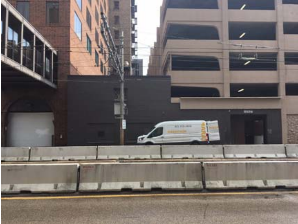
HE-MPC-12122, August 2018, primary facade, looking north
