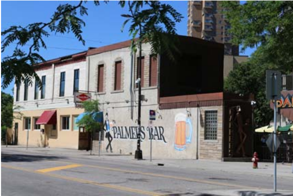
HE-MPC-4935, June 2018, primary facade, looking southwest
