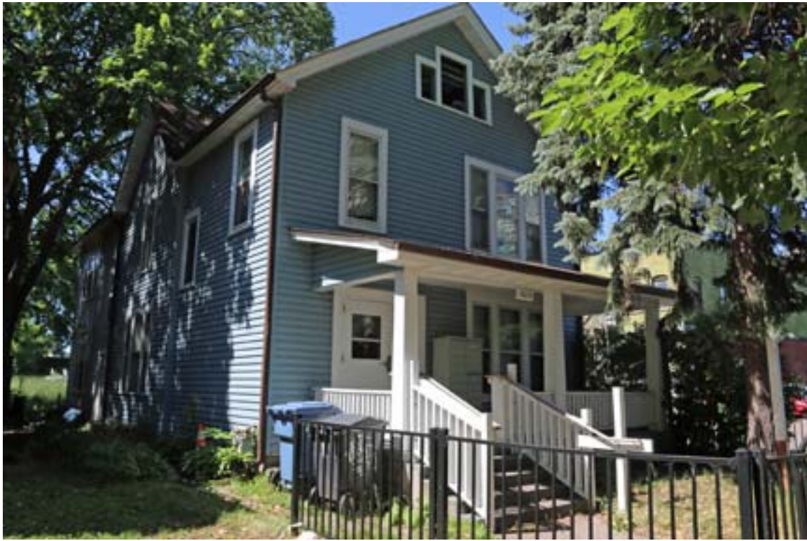
HE-MPC-19324, June 2018, primary facade, looking southwest
