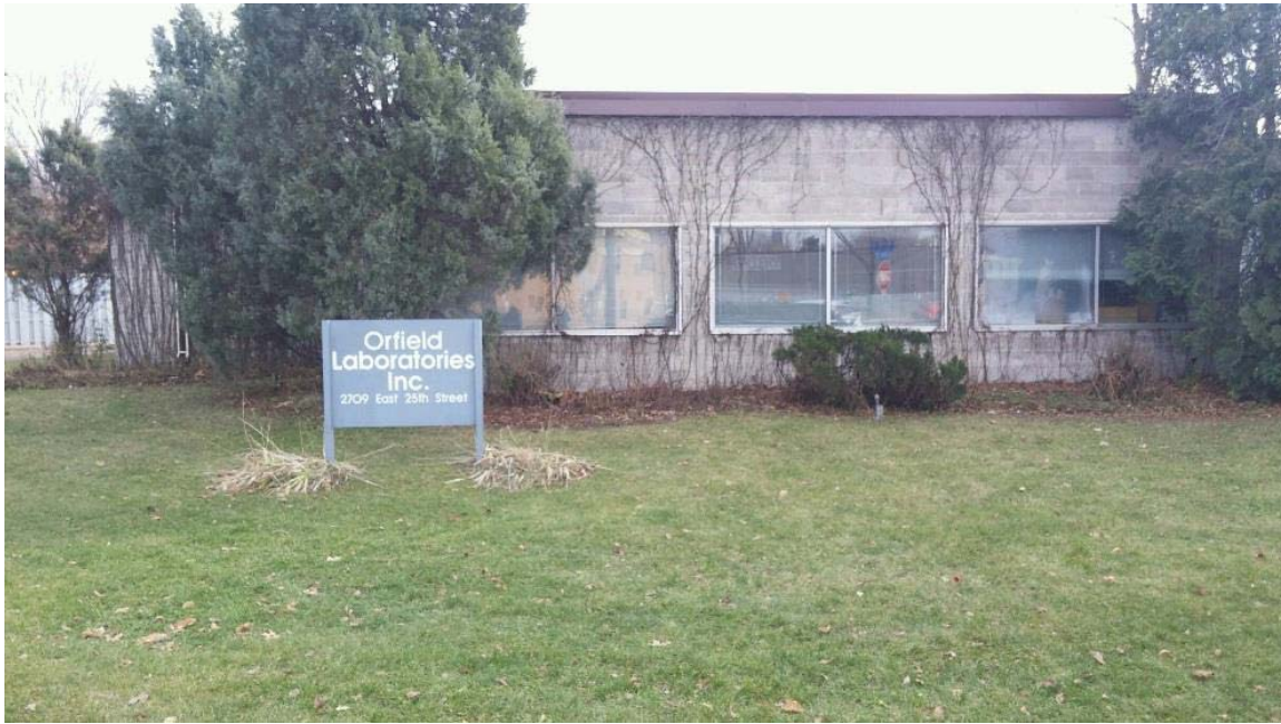
HE-MPC-3949, July 2018, primary facade, looking southeast
