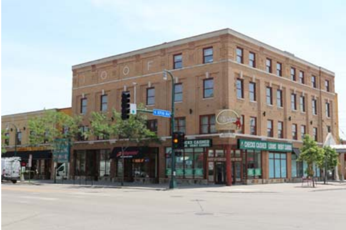
HE-MPC-7702, June 2018, primary facade, looking southeast
