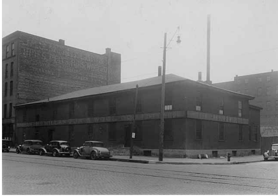
200 1 st Avenue North (1st Hall)
