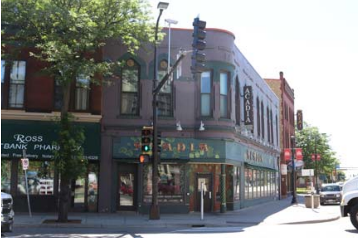
HE-MPC-4923, June 2018, primary facade, looking east
