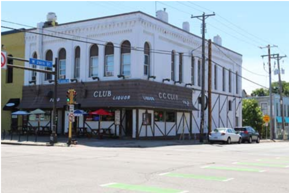
HE-MPC-19326, June 2018, primary facade, looking southwest
