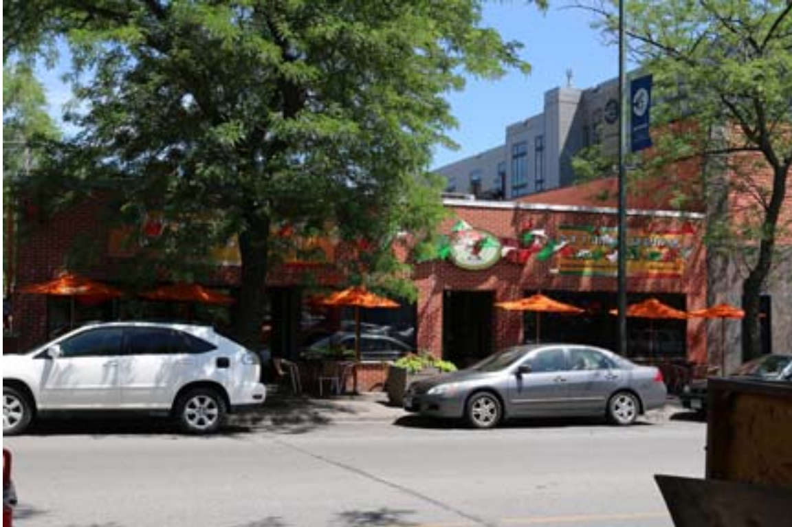
HE-MPC-12553, June 2018, primary facade, looking east
