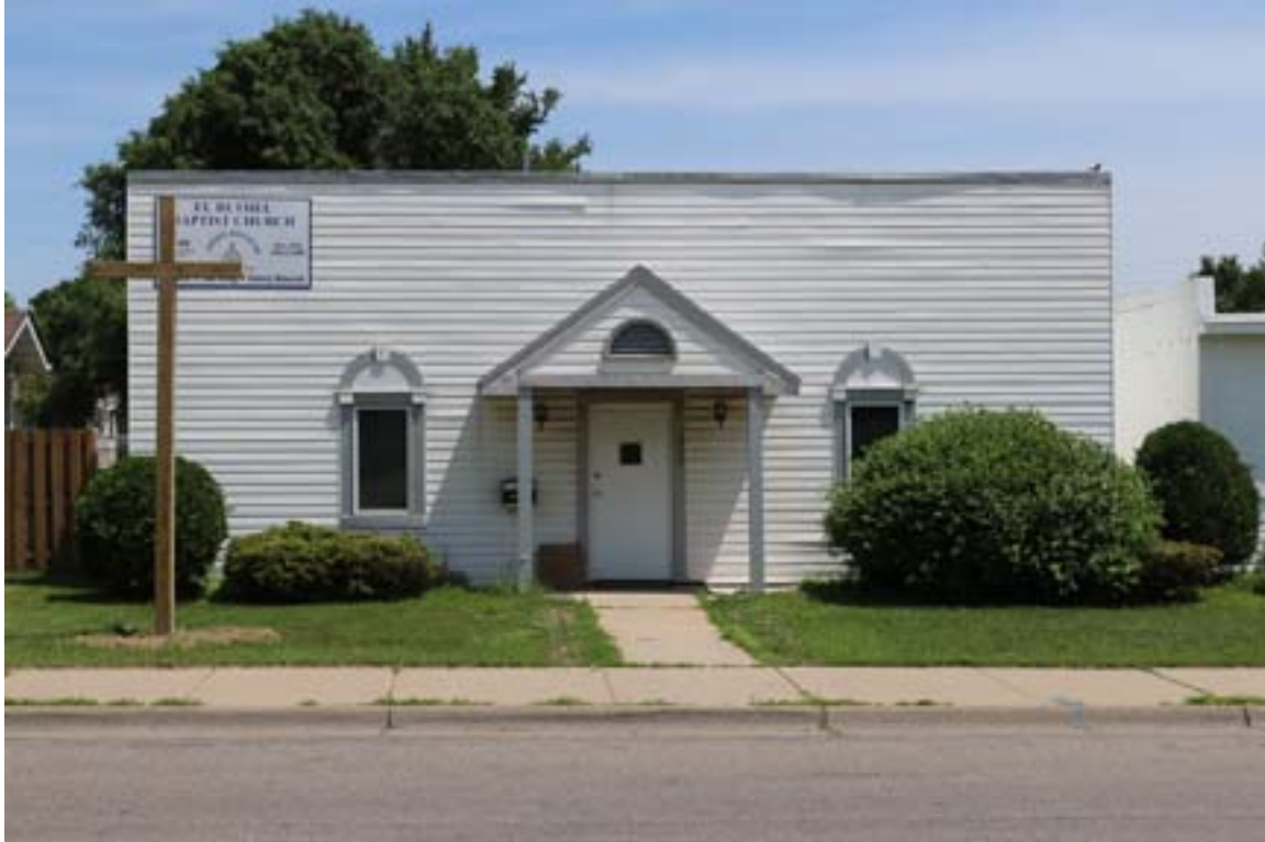
HE-MPC-4886, June 2018, primary facade, looking east
