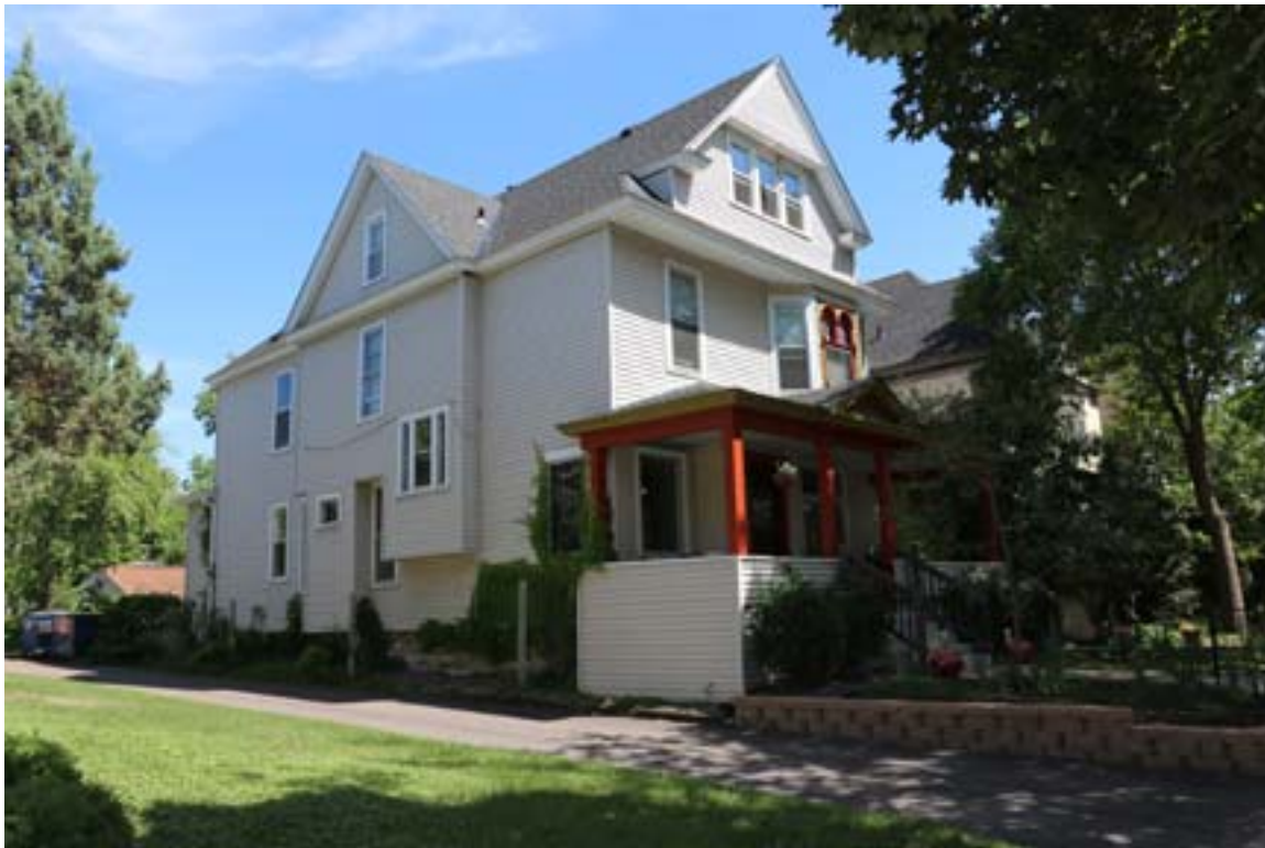
HE-MPC-19327, June 2018, primary facade, looking southeast
