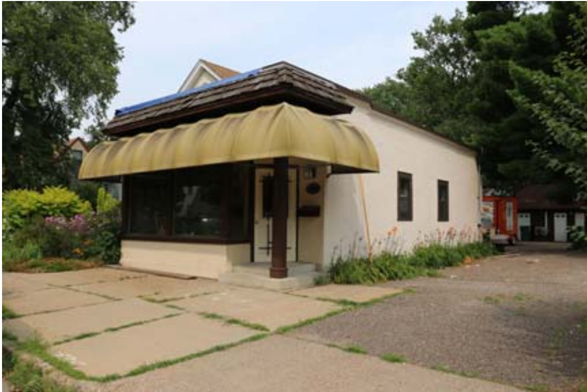
HE-MPC-19330, August 2018, primary facade, looking northeast
