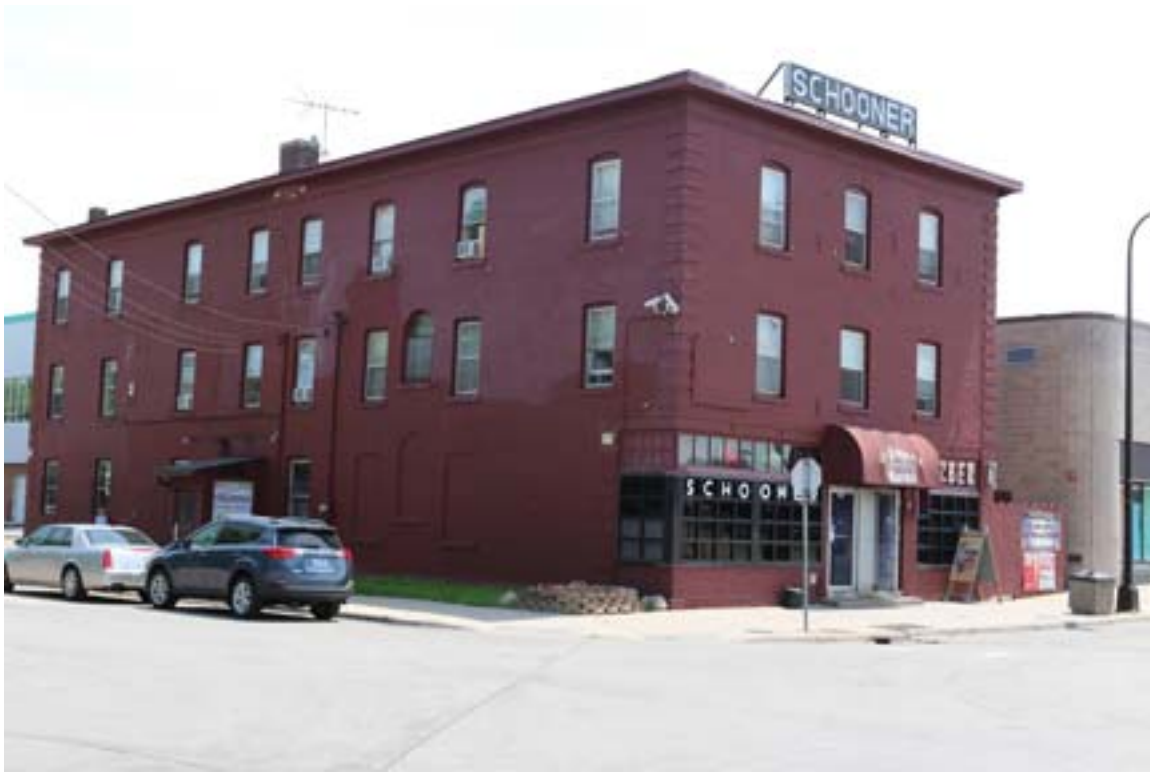
HE-MPC-3904, June 2018, primary facade, looking southeast
