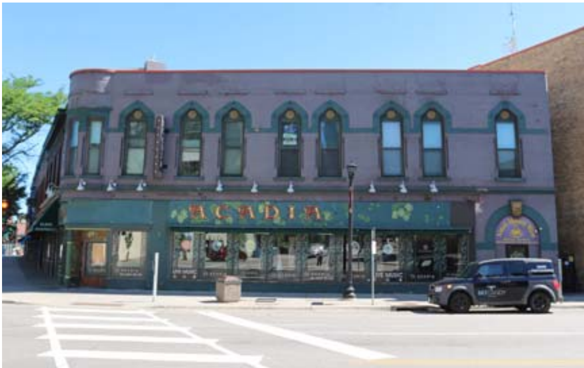
HE-MPC-4923, June 2018, primary facade, looking north
