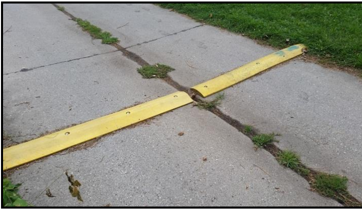
Figure F-22. Alley Speed Bump
