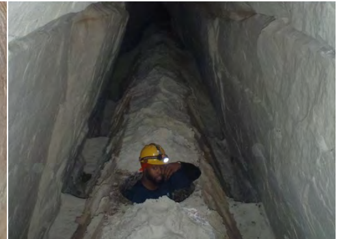
Void and sediment buildup in and around tunnel
