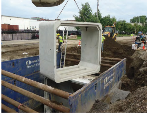
12x10 Infiltration Box Culvert Installation
