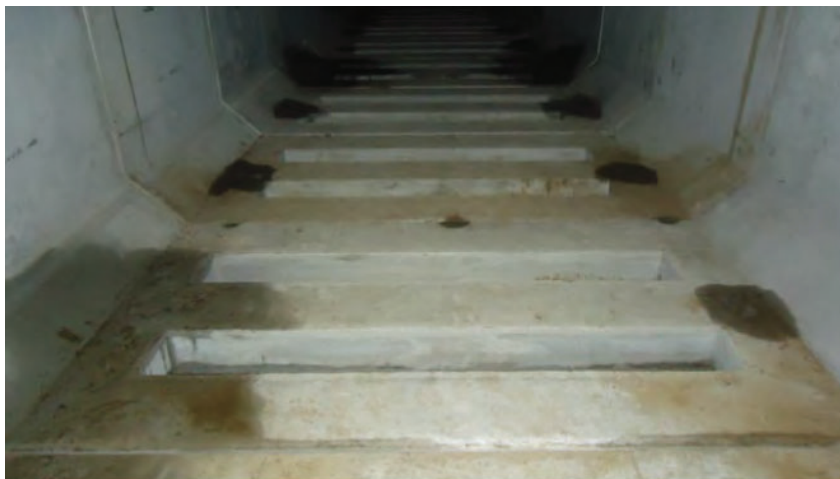
Infiltration Box Culvert – inside view
