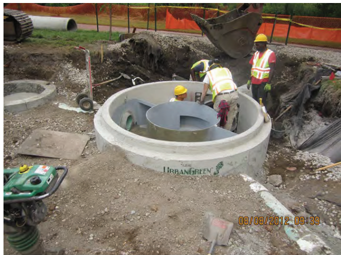
Grit Chamber Construction at Dean Pkwy
