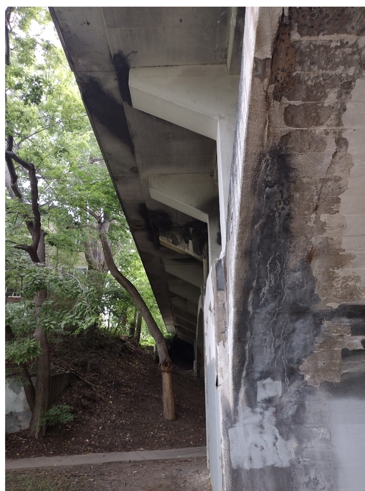
Additional photos of spalling concrete, exposed rebar, and existing bridge conditions.
