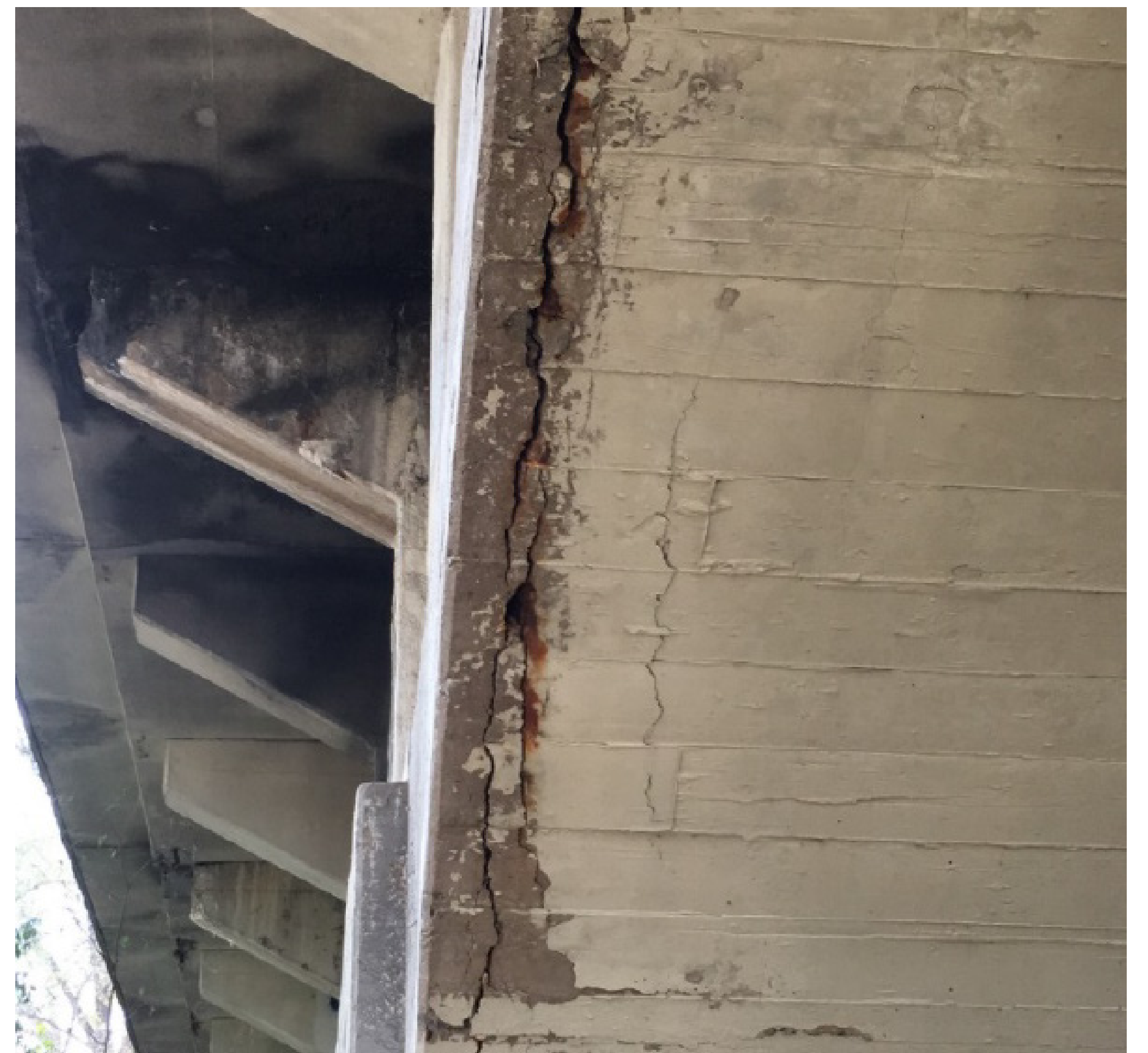
Cracks and Concrete Spalling on Arch Rib
