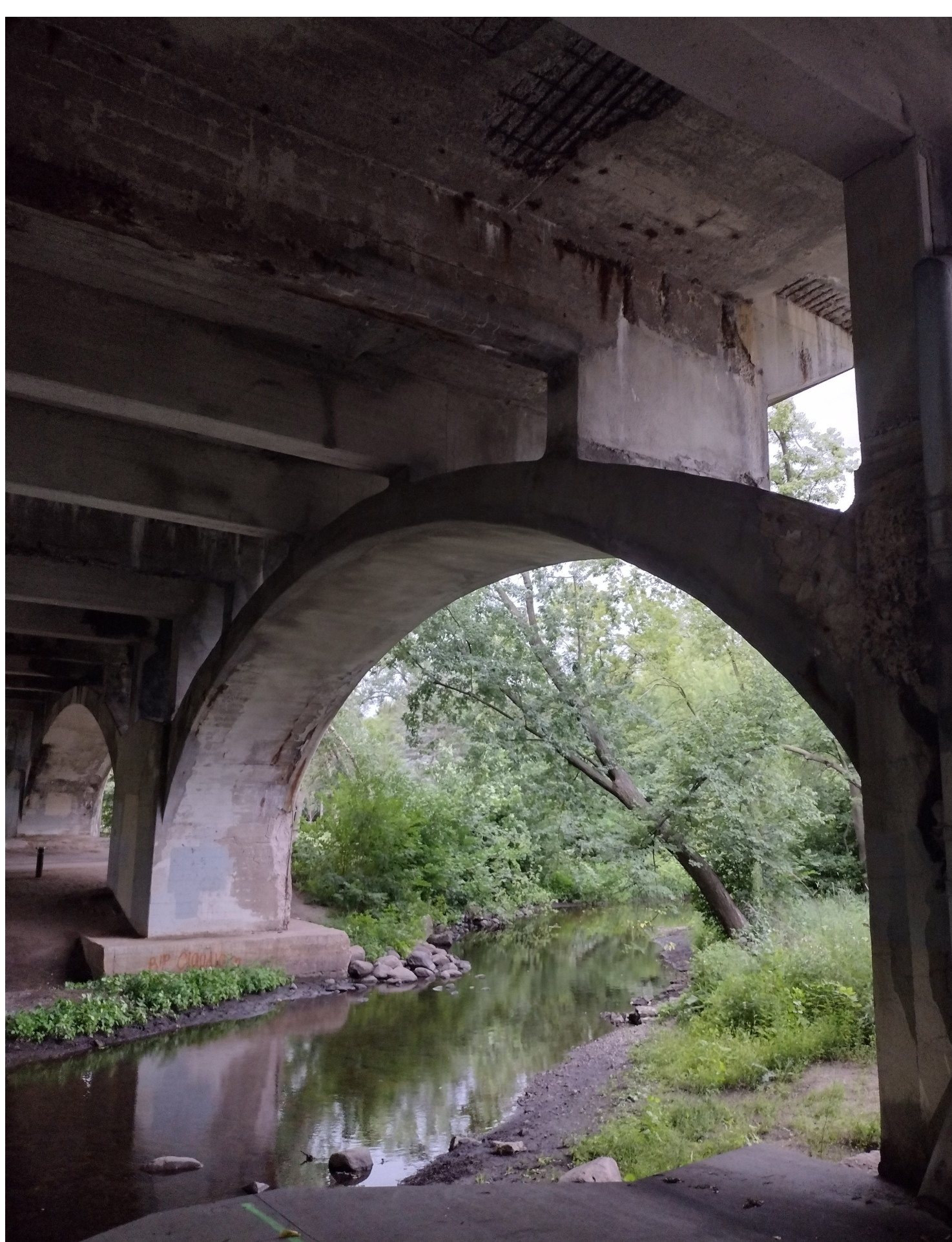
Additional photos of spalling concrete, exposed rebar, and existing bridge conditions.
