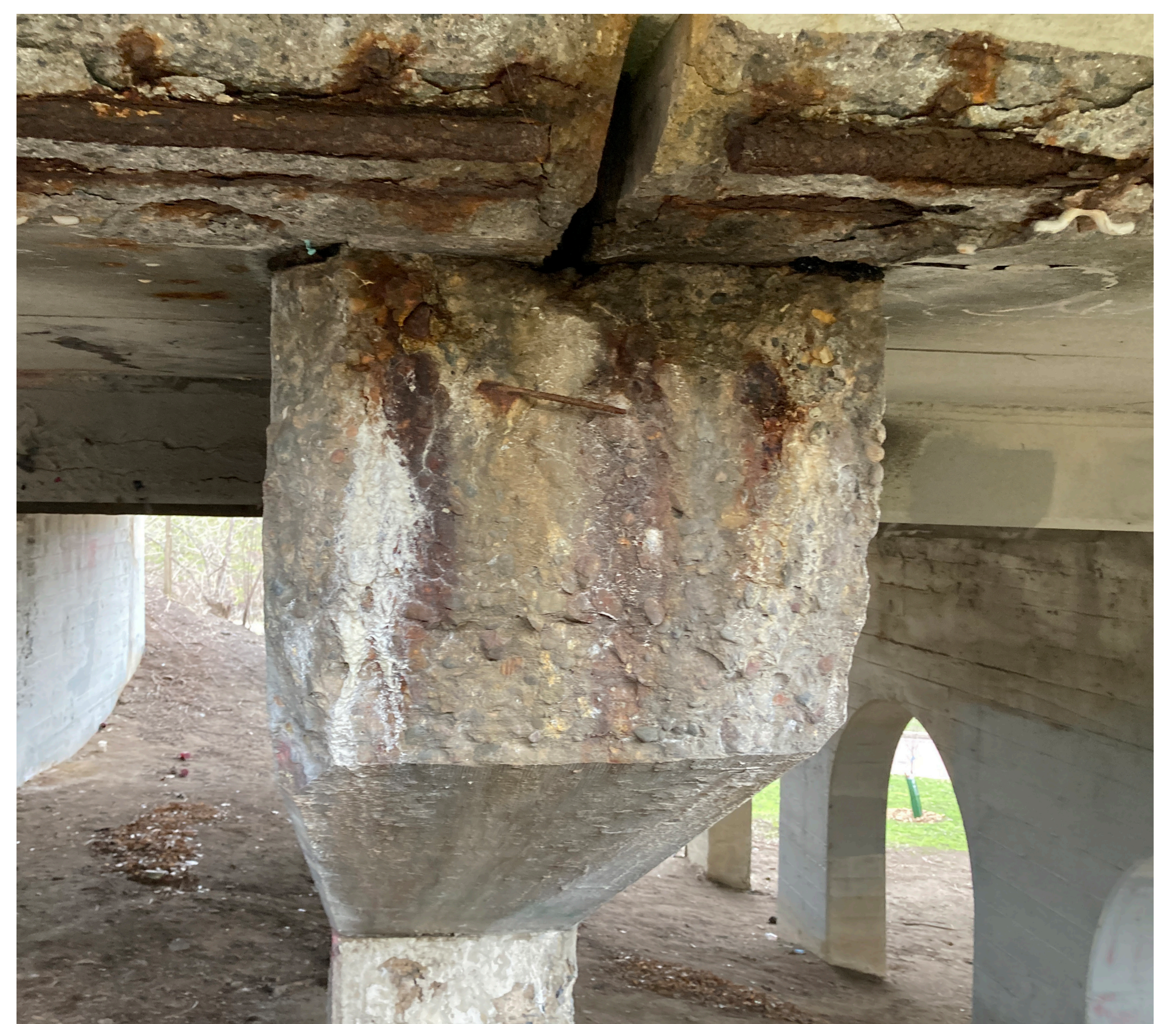
Cracks and Concrete Spalling on Arch Rib
