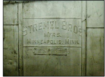
Fire door dating to the period of significance
