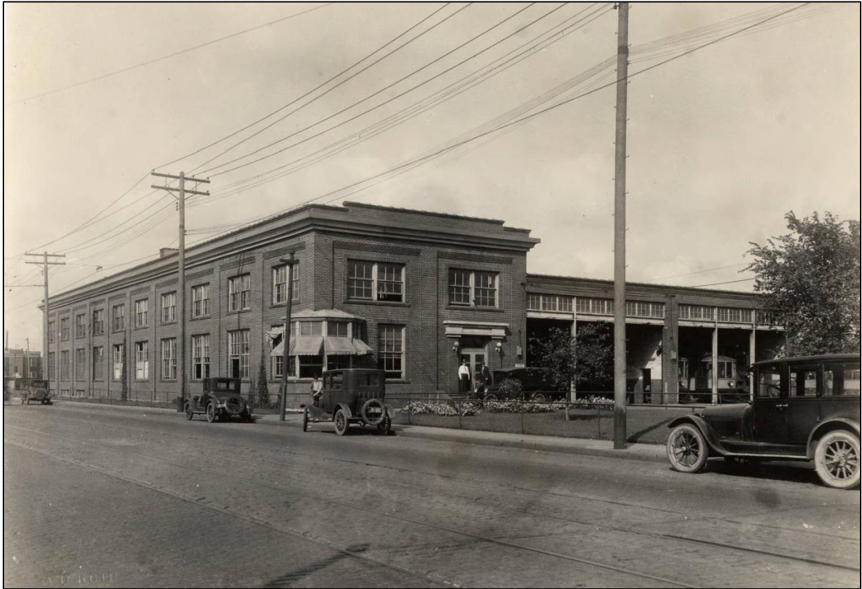
Figure 3. North Side Station 1922. Note the five-part bay window, the main entry, the shed car bays, the divided light windows and the open space in front of this part of the building. Any changes to the exterior of the 1914 building and any partial or complete demolition of the 1954 addition should move to restore the building back to this form. Source: Minnesota Streetcar Museum.
