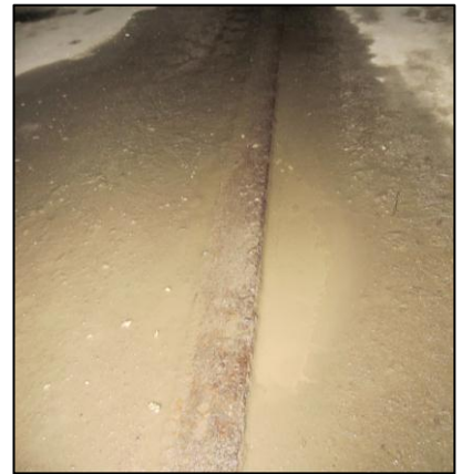
Exposed streetcar tracks in the former car sheds
