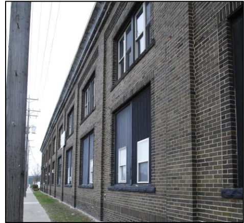
Infill panels and replacement windows.
