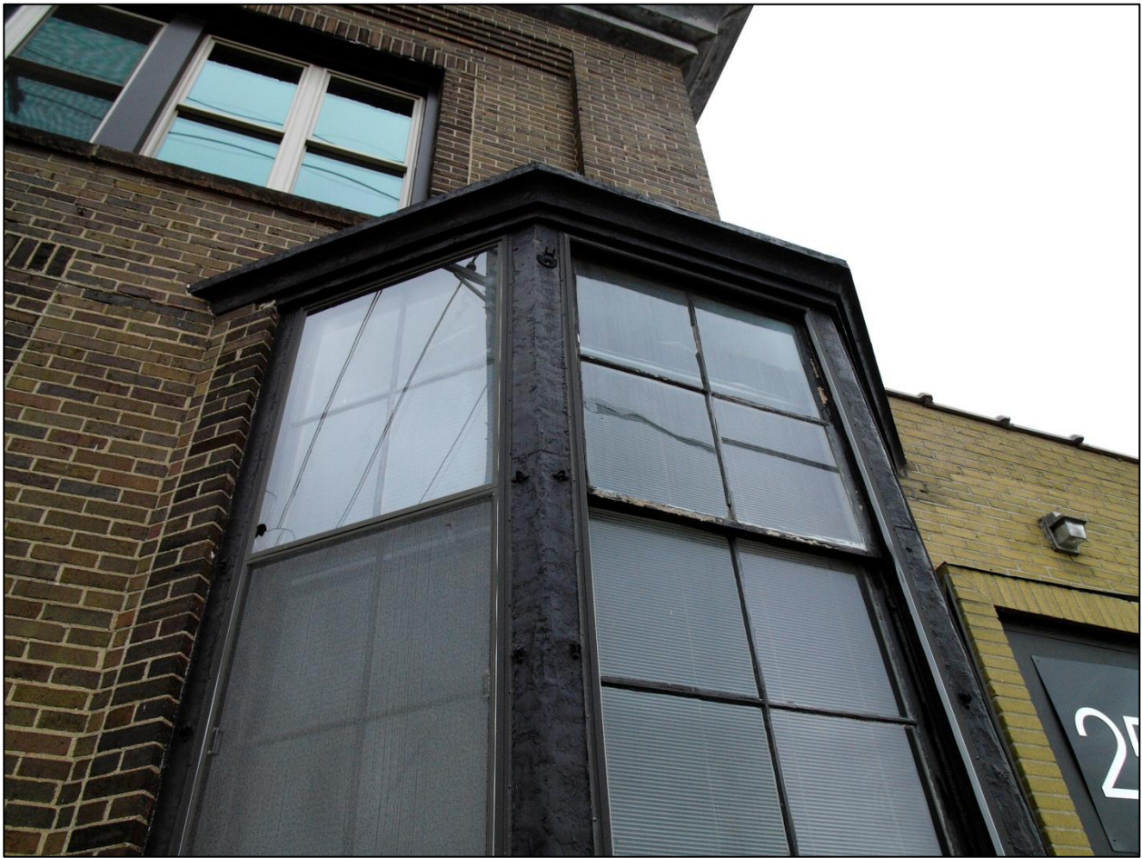
Figure 6. Portion of the five-part bay window that protrudes outside of the present entry. Source: CPED files.
