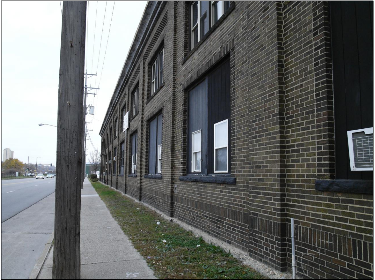
Figure 9. Infill panels and replacement vinyl windows on 1914 building. Source: CPED files.
