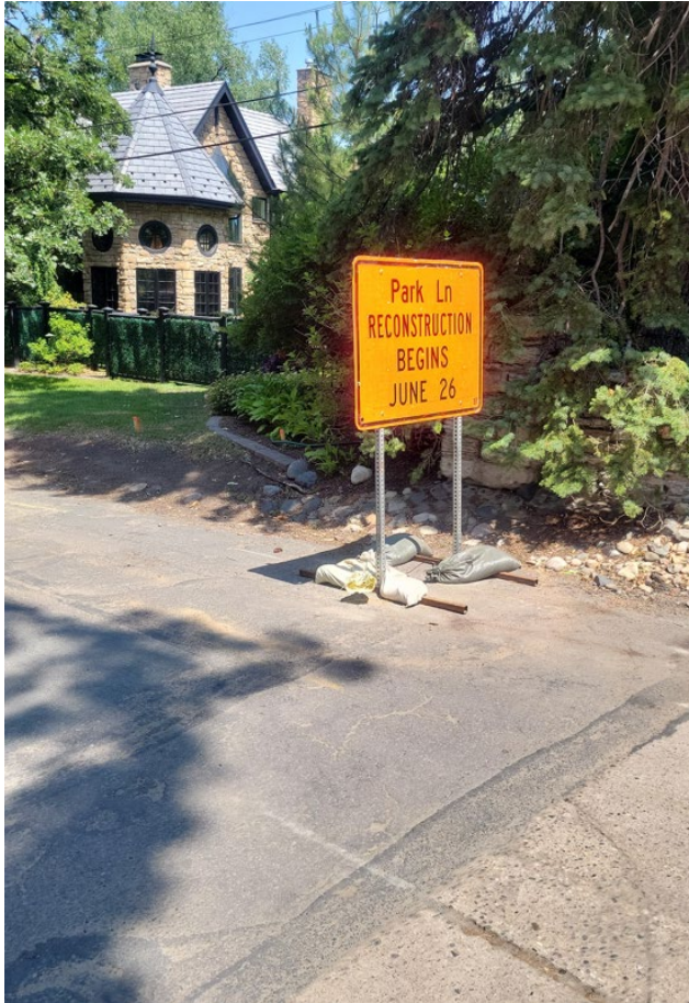
Advanced notice signage
