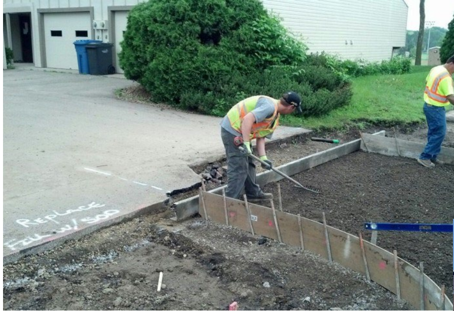
Forming and Pouring Driveways
