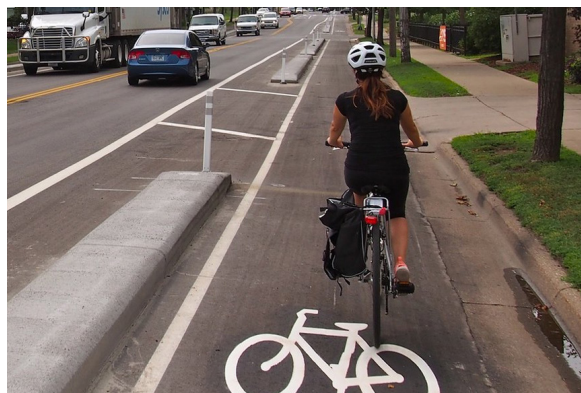
Curb Protected Bike Lanes
