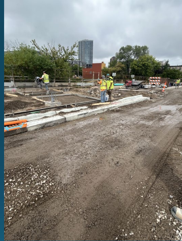
South of I-94 Bridge – Concrete Flatwork Preparation
