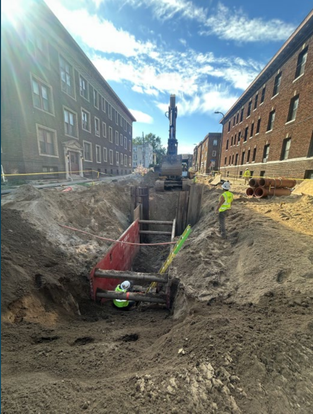
South of I-94 Bridge – Sanitary Sewer Installation
