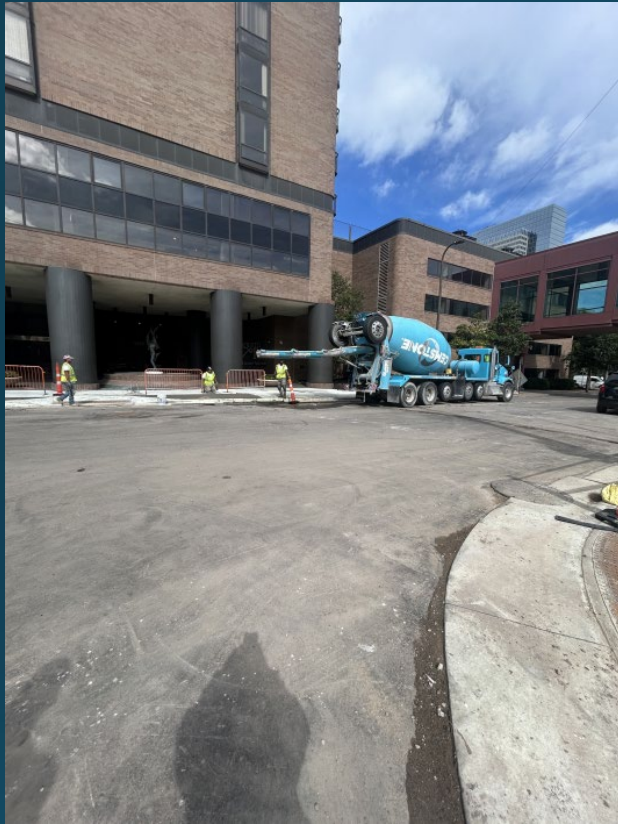
Grant St – Concrete Flatwork Installation
