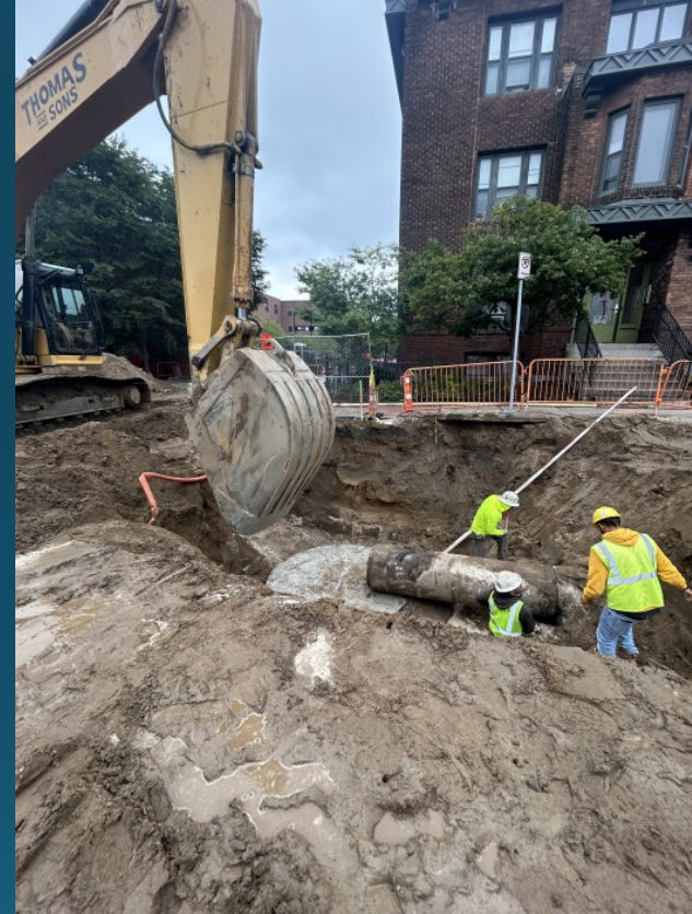
South of I-94 Bridge – Storm Sewer Installation
