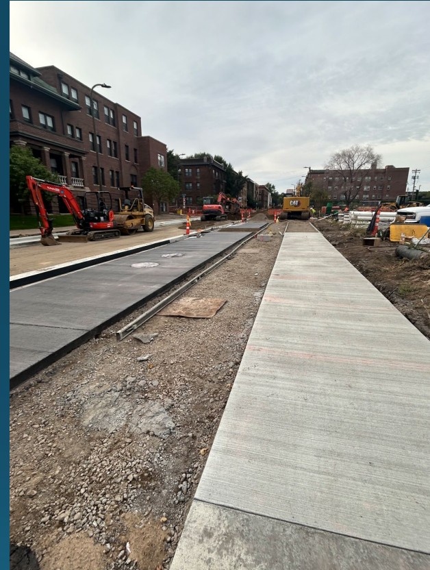
South of I-94 Bridge – Flatwork installation
