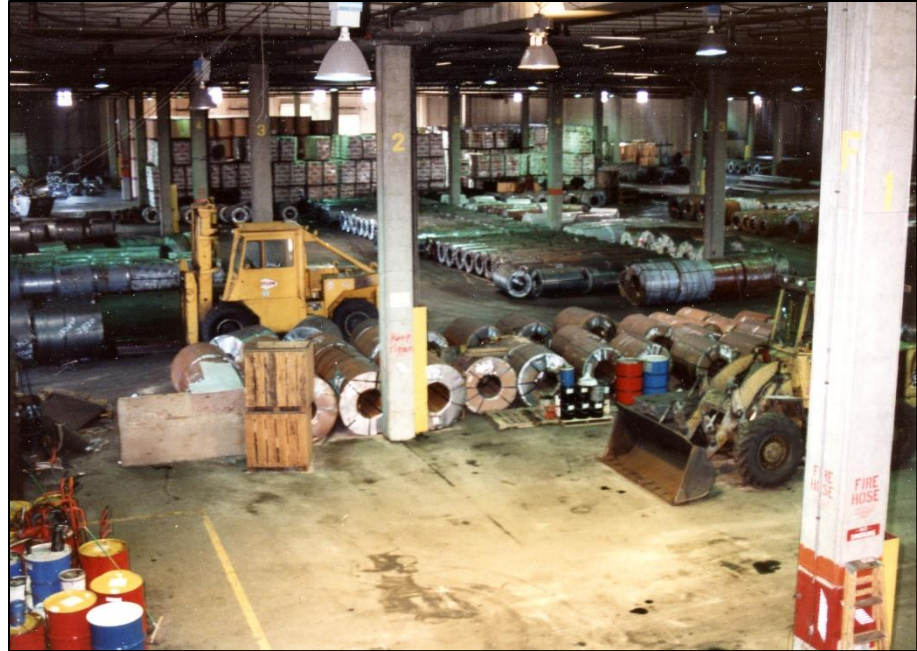
Warehouse interior, ca. 1985, looking south. (City of Minneapolis)
