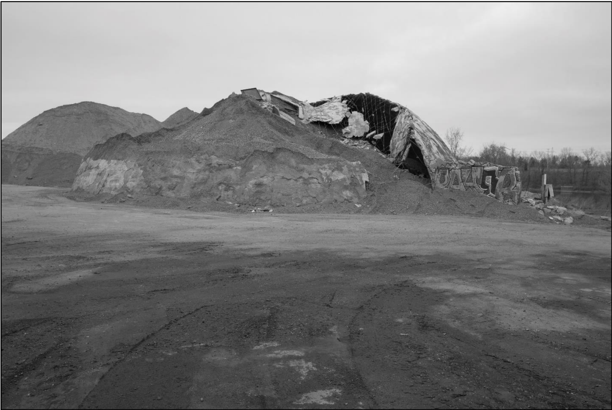
Dome, HE-MPC-9670, after collapsing, 2018. (City of Minneapolis)
