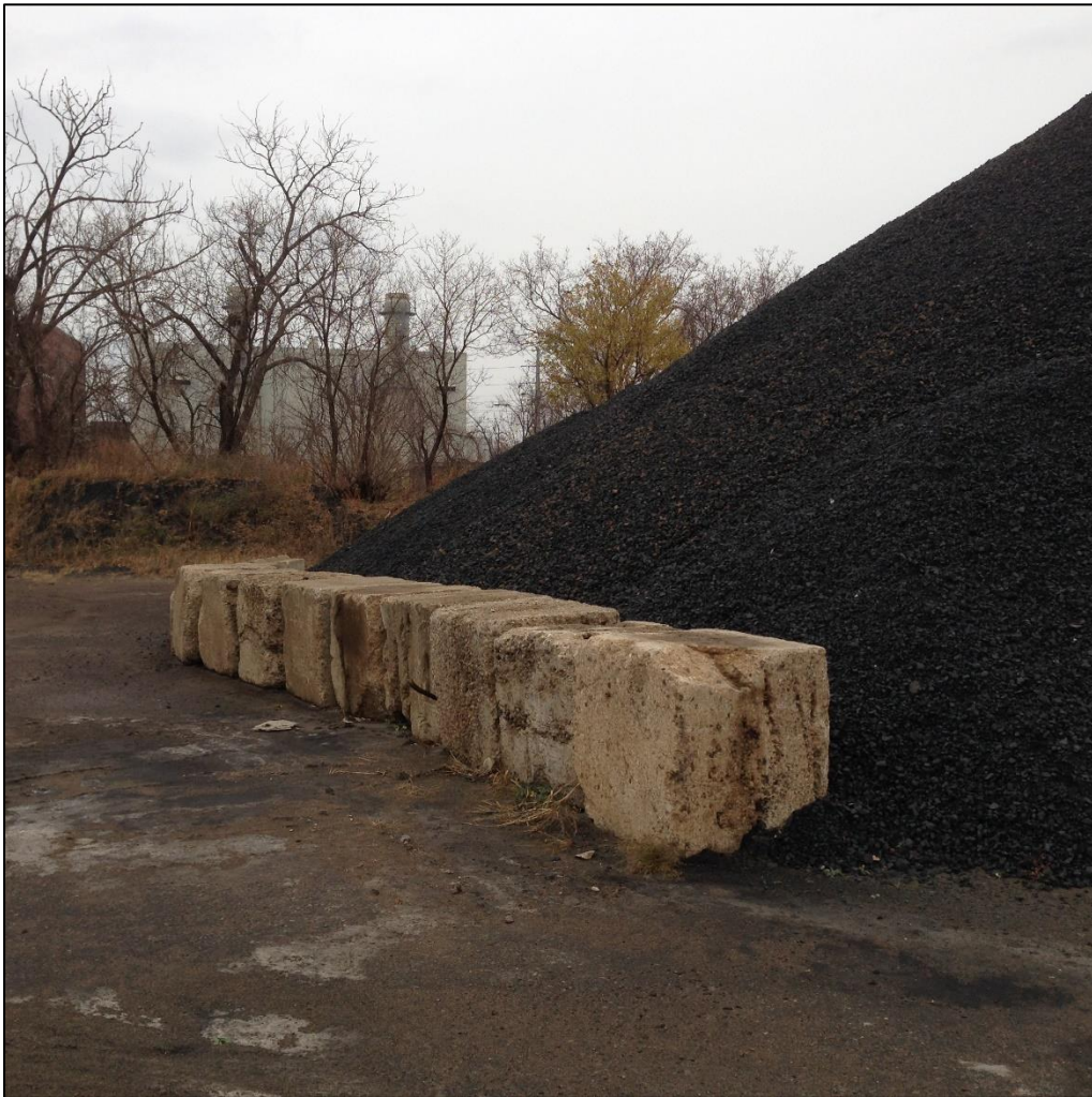
Concrete cubes holding back coal at the base of a commodities pile on the Upper Harbor Terminal, 2014. (Hess, Roise and Company)
