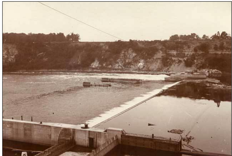
Constructing Meeker Island Lock and Dam on the Mississippi River near the Franklin Avenue Bridge, Minneapolis, ca. 1904. (Minnesota Historical Society)
