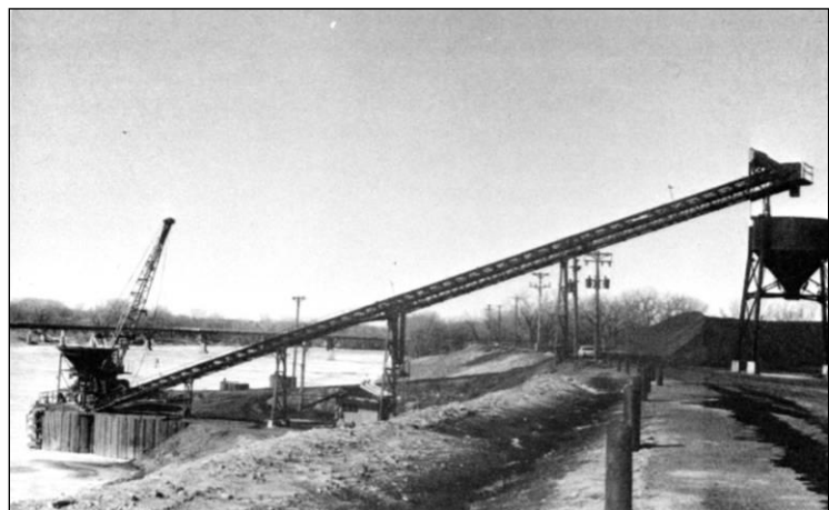
The NSP Riverside Station barge dock facilities, ca. 1968. (Merlin H. Berg, “Upper Harbor Terminal Report”)
