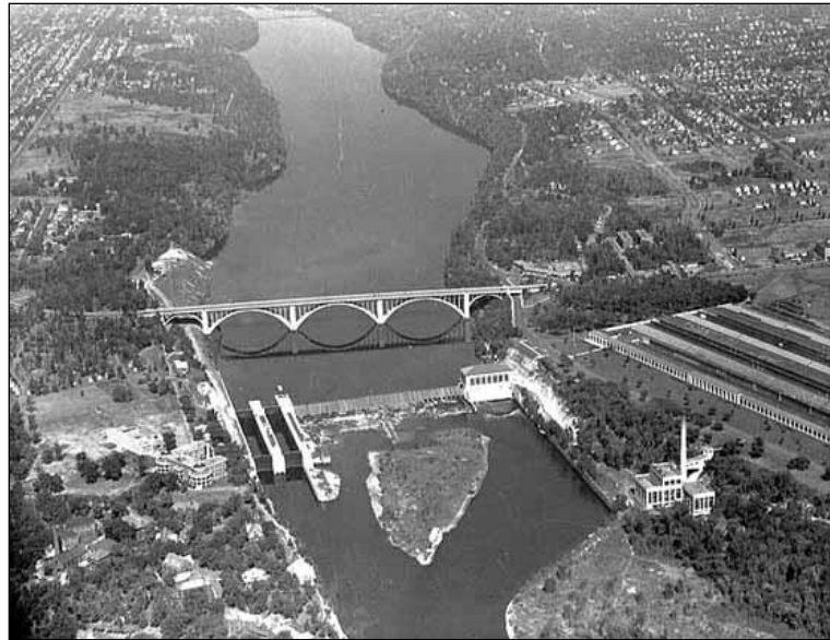
Government Lock and Dam No. 1, Saint Paul, 1936. The Ford Dam, as it is commonly known, provided a thirty-foot lift that rendered the Meeker Island dam obsolete. (Minnesota Historical Society)
