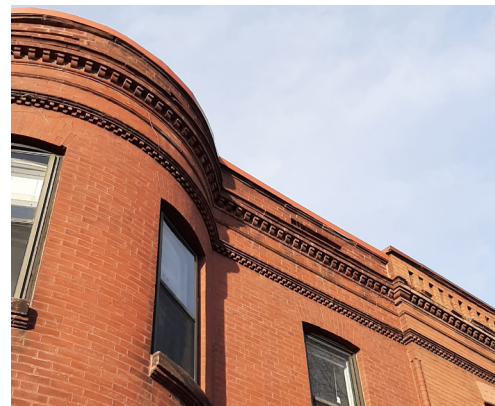
Note the historic brickwork at 100 25th St E. These rowhouses have brick dentils and brackets along the cornice line.
