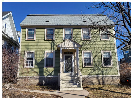
Built in 1998, the house at 2515 1st Ave S has a masonry foundation and one cladding material. The windows have divided lights.
