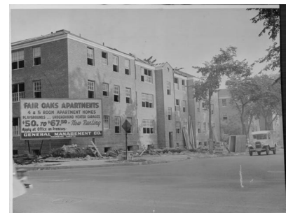
The Fair Oaks Apartments at 2421 3rd Ave S, built in 1939, were the last to be built during the period of significance. Courtesy of the Hennepin County Library James K. Hosmer Special Collections.
