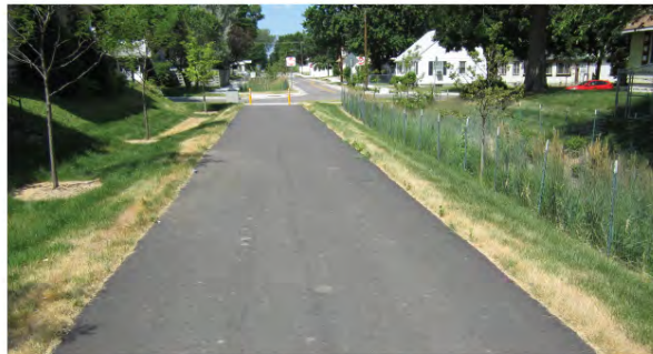
Rain gardens along the completed 37th Ave Greenway provide water quality benefits. Flood storage is located under the mixed-use trail.
