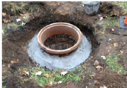
Infiltration & Inflow Repairs
