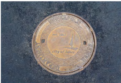
Manhole Cover Replacement
