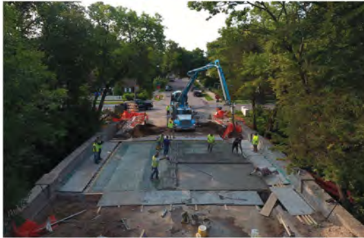
Bridge repair and rehabilitation underway
